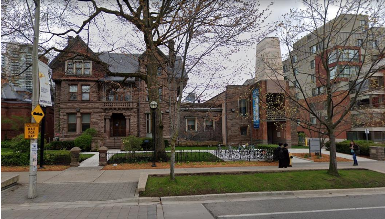
Detail of the Alexander McArthur House (left) and the KPMB & Barton Myers Associates Inc. tower addition (right)
