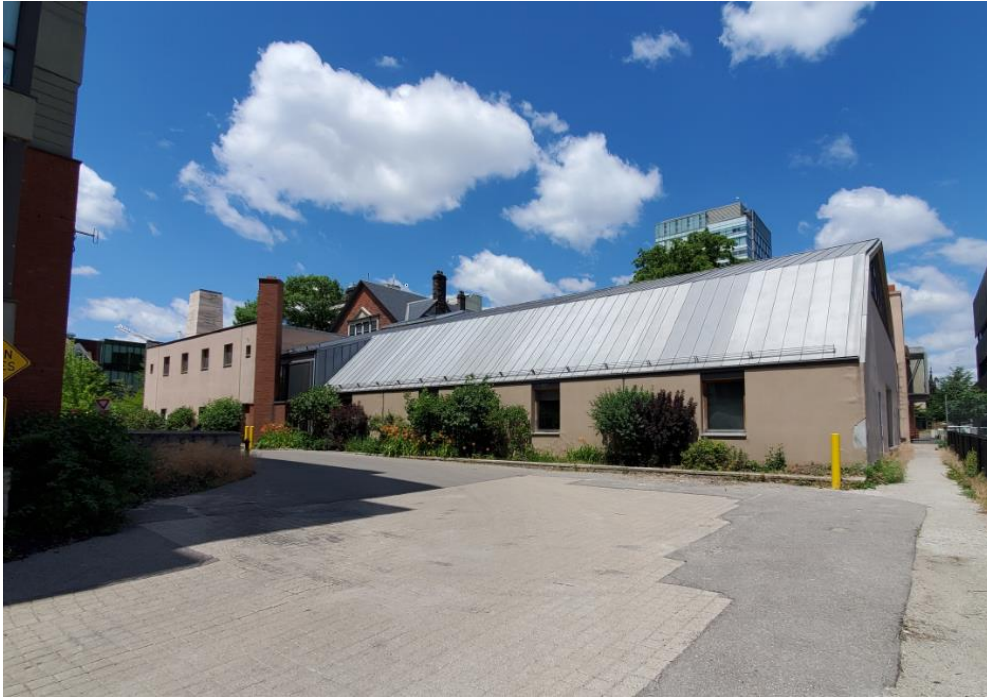
Detail of the former Drill Hall
