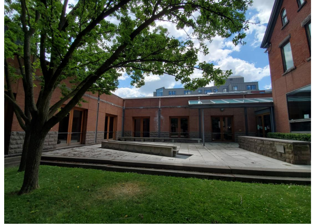
Detail of the L-shaped KPMB & Barton Myers Associates Inc. addition at the rear and the Peter F. Bronfman Courtyard looking south
