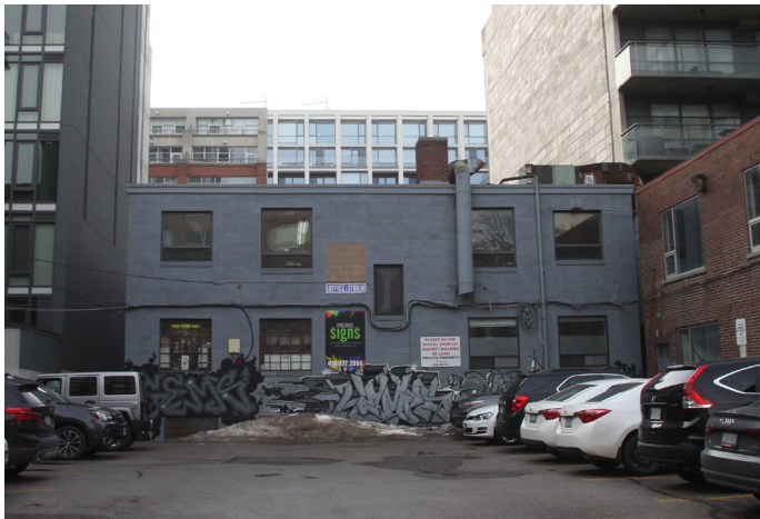
3. View of the north (rear) elevation of 38 Camden Street (March 14, 2019)
