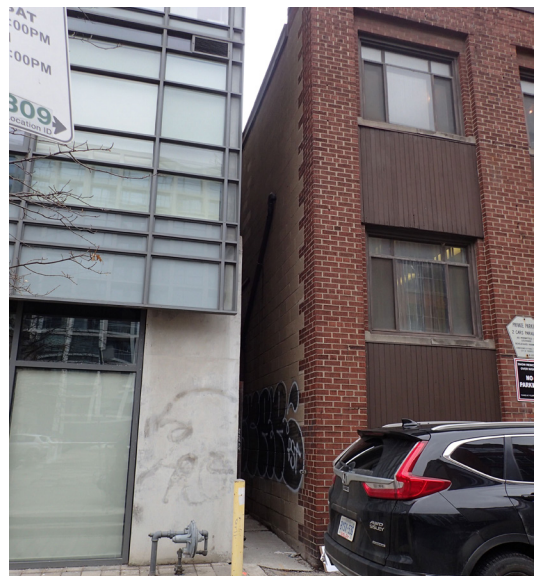
4. View of the west elevation of 38 Camden Street (March 15, 2019)
