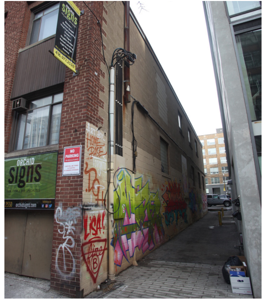
2. View of the east elevation of 38 Camden Street (March 14, 2019)
