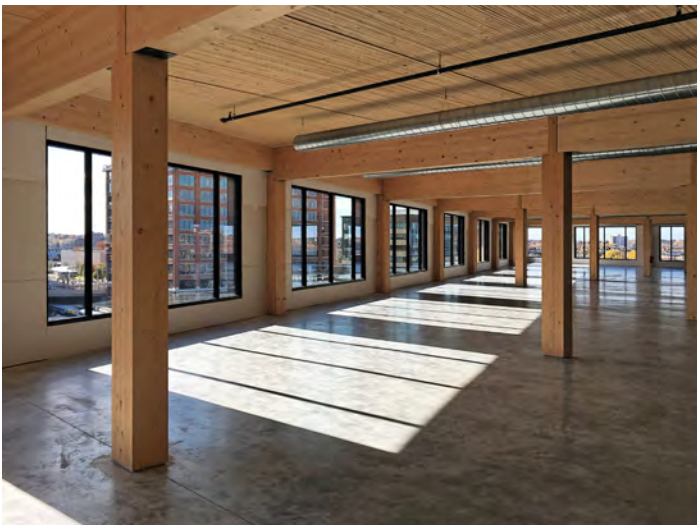
The T3 Building in Minneapolis is a 7 storey building made of heavy timber and nail laminated timber, which results in a flexible floor plate. Post and beam construction avoids shear walls, which maximizes flexibility over time.
