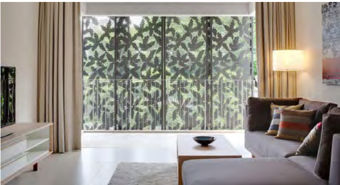
The private balcony of a unit in Kent Vale, Singapore animates the living room with a movable perforated metal screen incorporated into the building facade. The screen provides safety and the ability to control sunlight.
