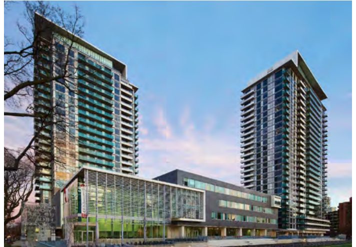
The North Toronto Collegiate Institute is integrated into the base of two residential towers. School amenities, including a theatre, classrooms and sports fields, are available to the community outside of school hours.
