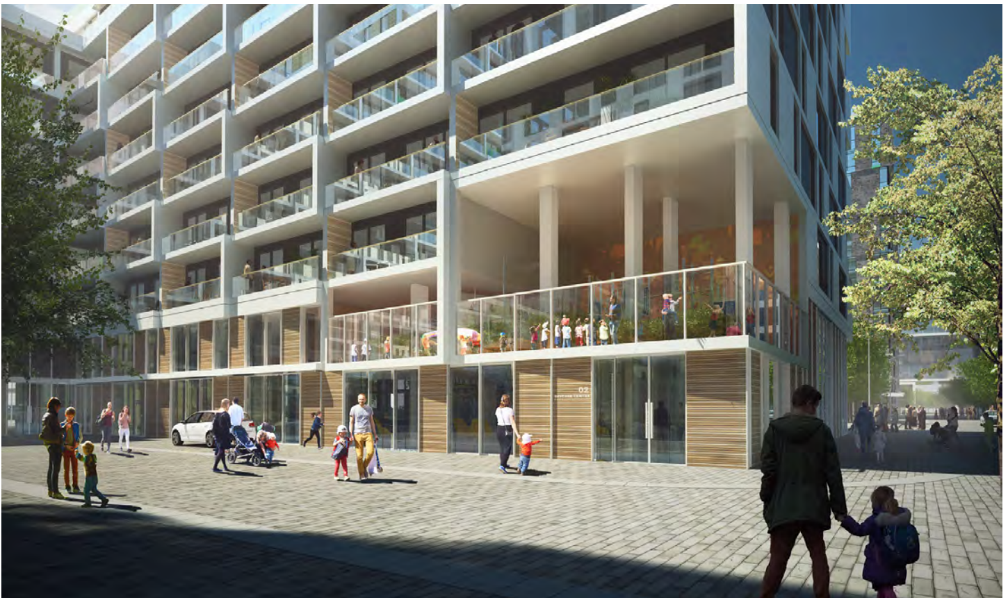
The Bayside development in Toronto shows how the child care's outdoor space was located on the 2nd level by taking a 'bite' out of the building. The covered outdoor space has the advantage of weather protection. Design features can also be added to bring light to darker areas of the space. This alternative massing solution was a response to a constrained site and involved cooperation between the developer (Waterfront Toronto), City Planning and Children Services.
