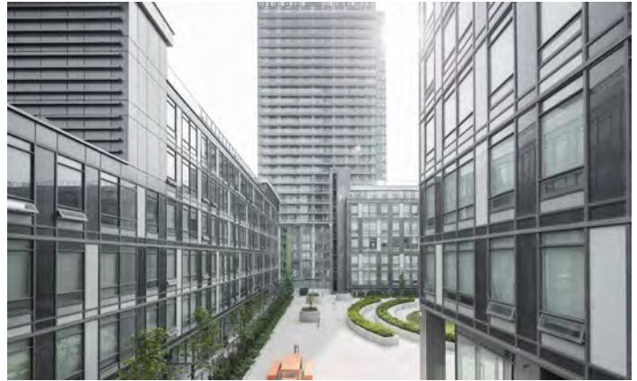
The third level of 150 Dan Leckie Way in Toronto opens onto a rooftop amenity space that features a variety of play spaces including a lawn and splash pad. Some units flow out into the space while others can informally supervise from above.
