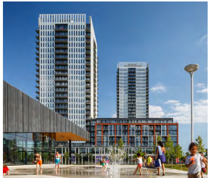
Regent Park is a phased, master planned community in Toronto with generous public facilities that anchor the public realm and animate the neighbourhood in all seasons. The central park and the pool facility were delivered in early phases.
