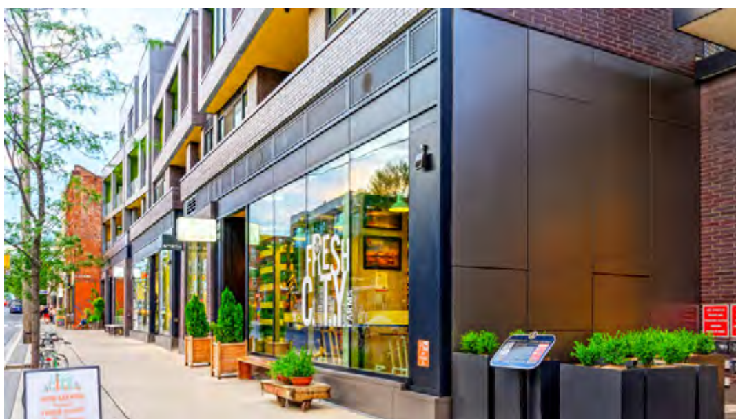
Venting and other base building services integrated into the base building frame around the façade.
