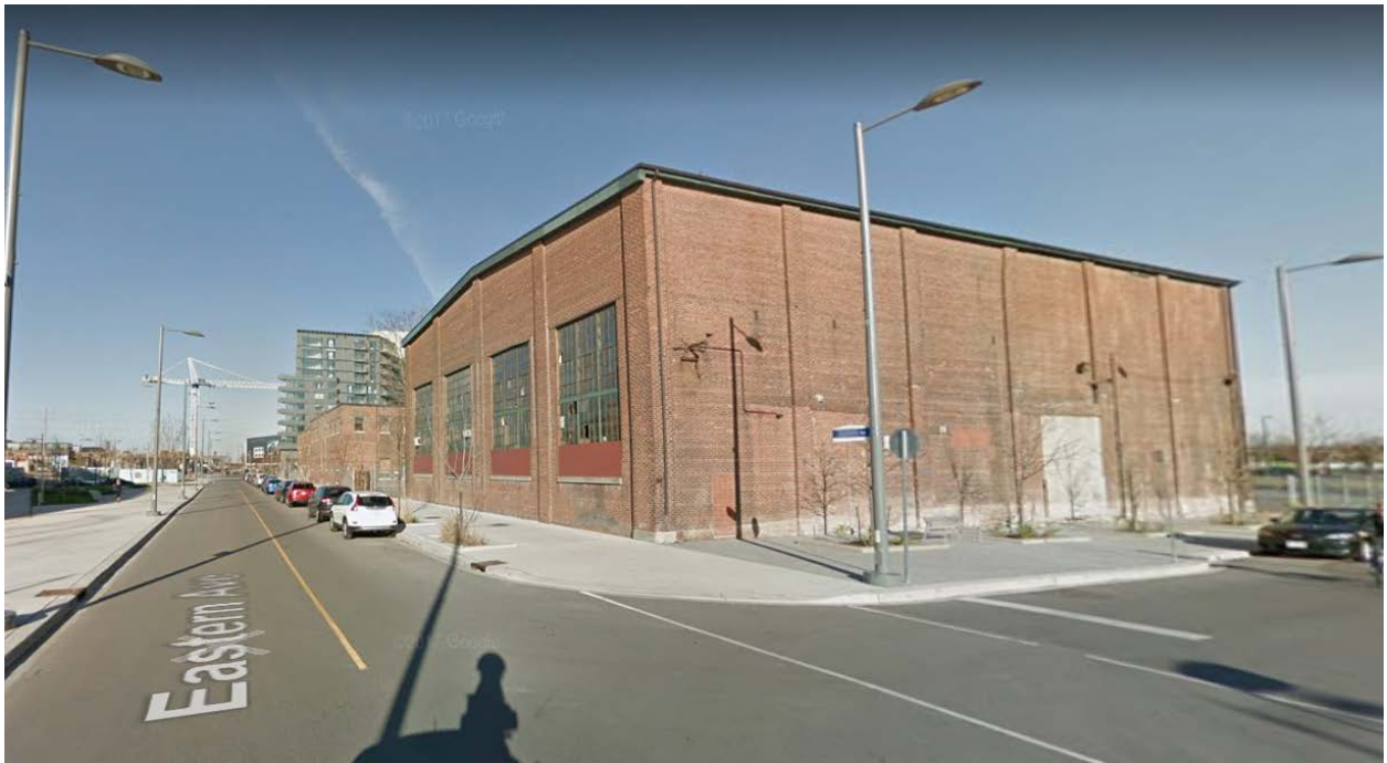
View looking southeast of 135 Eastern from Eastern Ave and Rolling Mills Road
