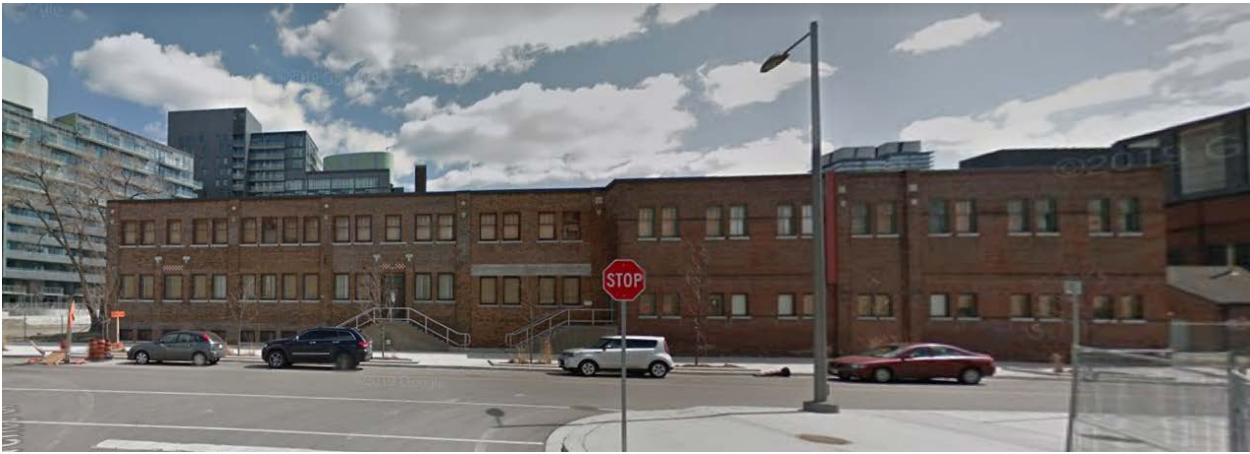
View looking south from Eastern Avenue and St Lawrence Street
