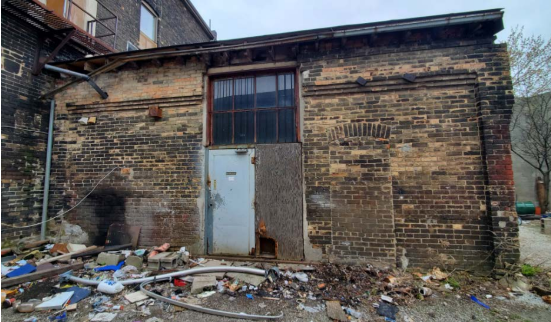
Figure 16. Detail of the ornamented parapet in the side (north) elevation of the rear one-storey brick building at 10A Dawes Road (Heritage Planning, 2021)
