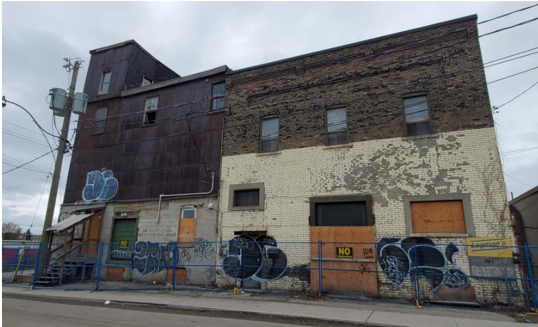
Figure 11. Detail of the principal (east) elevations of 10 (left) and 10A Dawes Road (right) (Heritage Planning, 2021)
