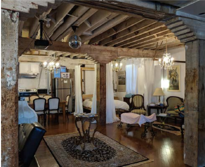
Figure 21. Detail of the ground floor of 10 Dawes Road illustrating the timber columns (ERA, 2018)
