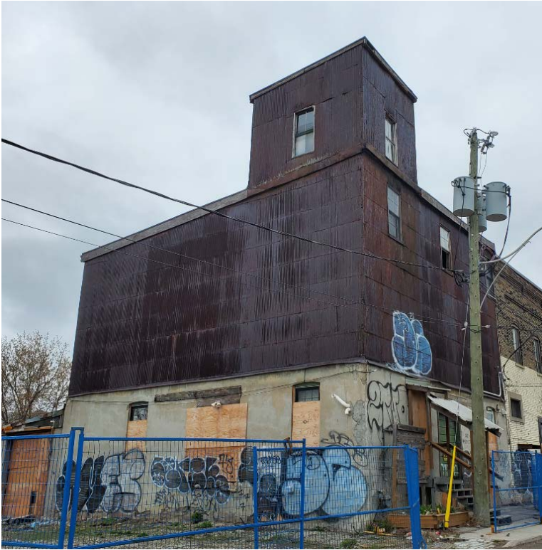
Figure 18. Detail of the southeast corner of 10 Dawes Road (Heritage Planning, 2021)
