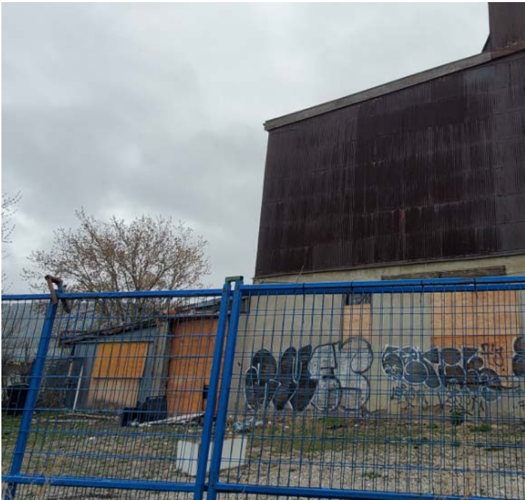
Figure 19. Detail of the one-storey concrete block addition and a one-storey metal clad addition at the rear of 10 Dawes Road (Heritage Planning, 2021)
