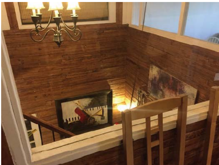
Figure 23. Details of the upper storeys at 10 Dawes Road where the 9 wooden-cribbed grain silos are (ERA, 2018)
