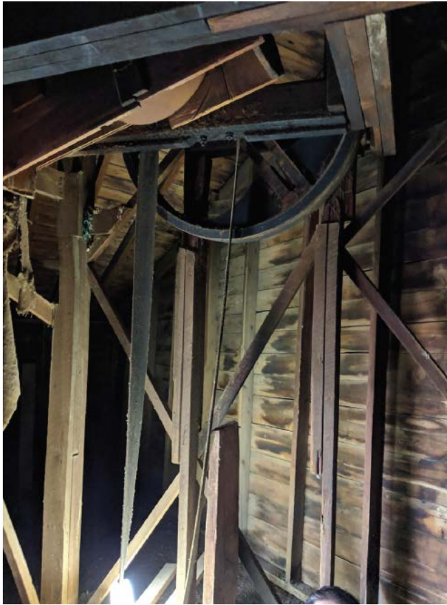
Figure 24. Detail of the original wheel and rubber conveyor belt still housed in the headhouse (ERA, 2018)
