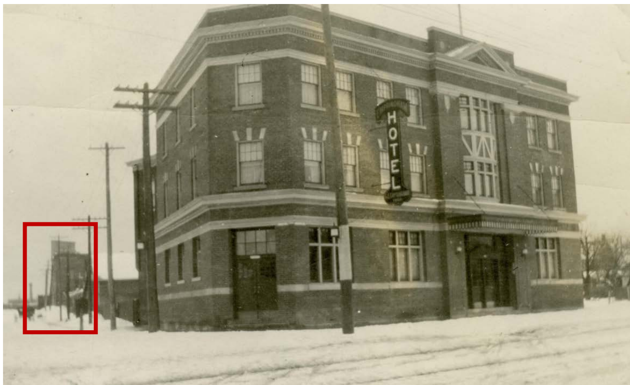
Figure 9. 1914 historical photograph showing the new Empringham Hotel, annotated to show the grain elevator at 10 Dawes Road in the background ( Toronto Public Library )
