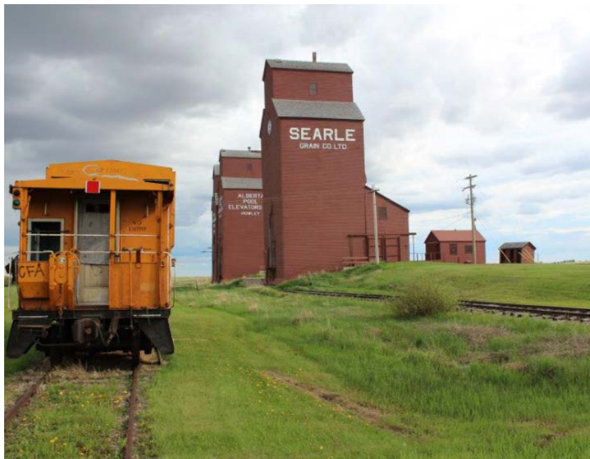
Figure 27. Example of a grain elevator, Alberta Wheat Pool Grain Elevator, Big Valley, Alberta (1960) (Heritage Planning, 2013)
