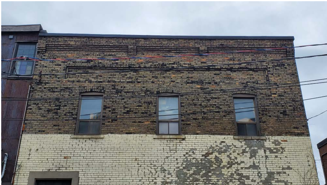
Figure 15. Detail of the ornamented parapet and inaid rectangular panel in the principal (east) elevation of 10A Dawes Road (Heritage Planning, 2021)
