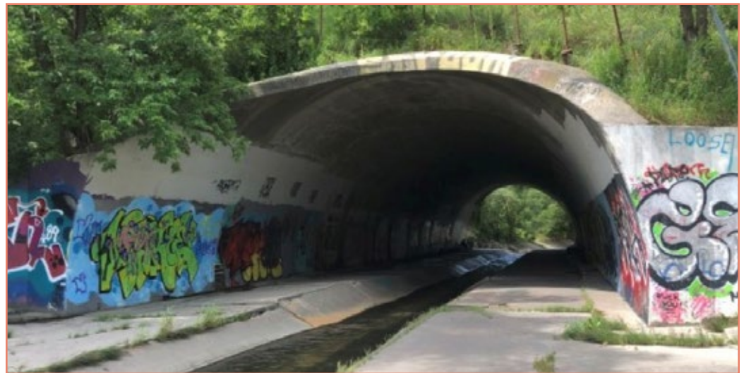
Example of a Culvert in Fair Condition – ID 091 Jane St over Black Creek
