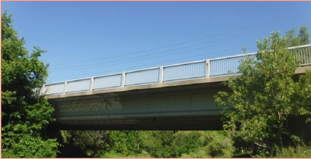
Example of a bridge in fair condition – ID 336 Steels Ave over Rouge River
