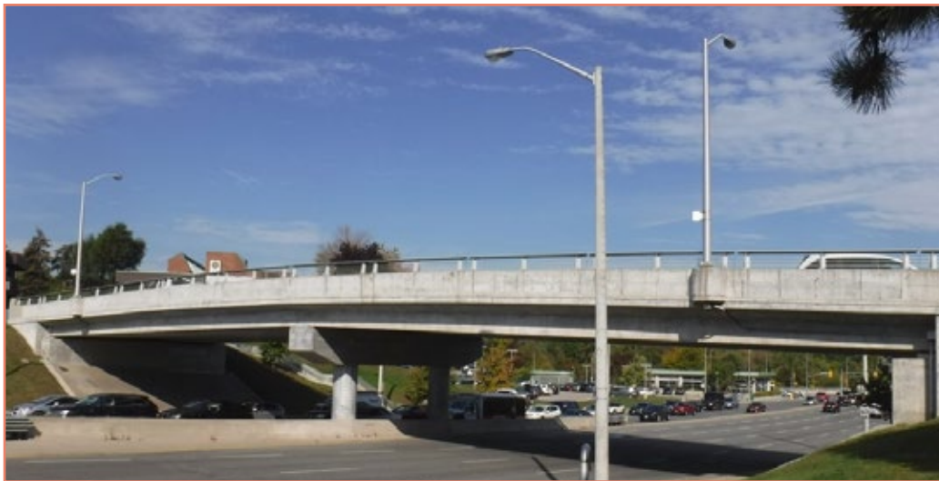
Example of a bridge in Good Condition – ID 250 Leslie under Old Leslie Hospital Ramp
