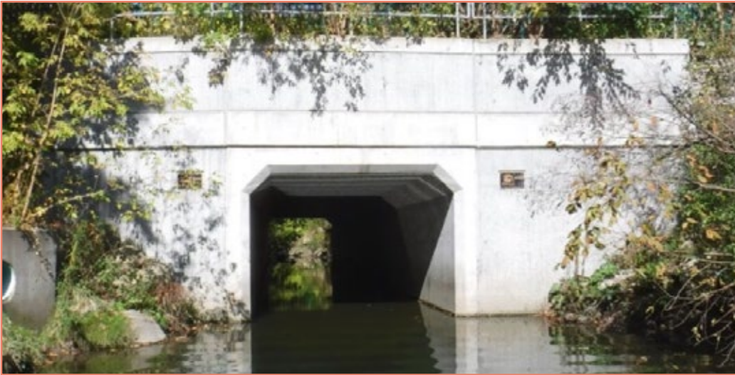
Example of a Culvert in Good Condition – ID 284 Lawrence Ave over Wilket Creek
