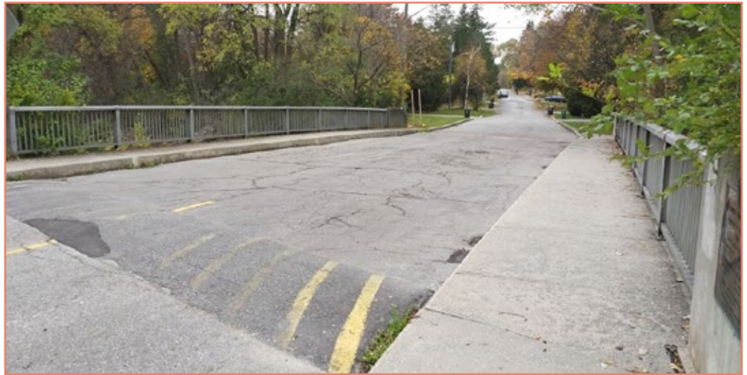
Example of a bridge in Poor Condition – ID 758 Don River Blvd over Don River
