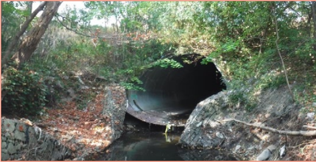
Example of a Culvert in Poor Condition – ID 267 Albion Rd over Albion Creek
