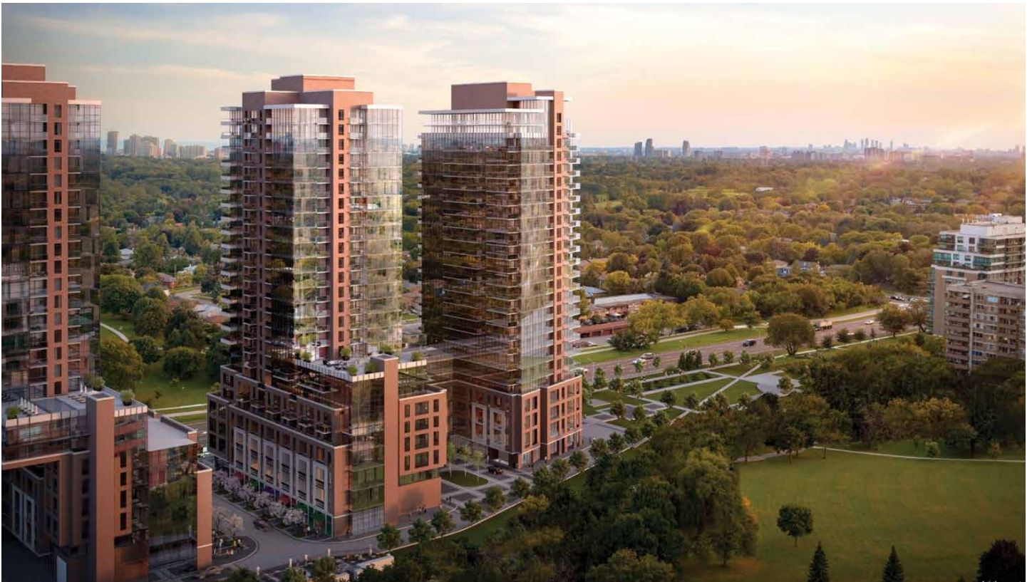
Figure 1. View of site facing south-west toward Eglinton Ave W.
