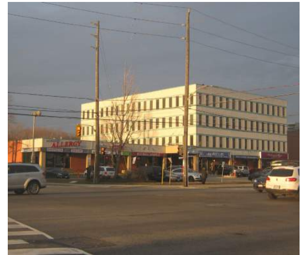
Northeast corner of Shaver Avenue South and Dundas Street West
