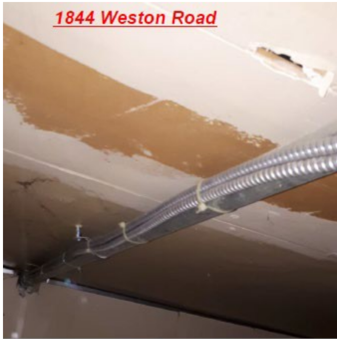
LOOKING UP INTO CEILING SPACE. EVIDENCE OF CRUMBLING DRYWALL ON CEILING.
