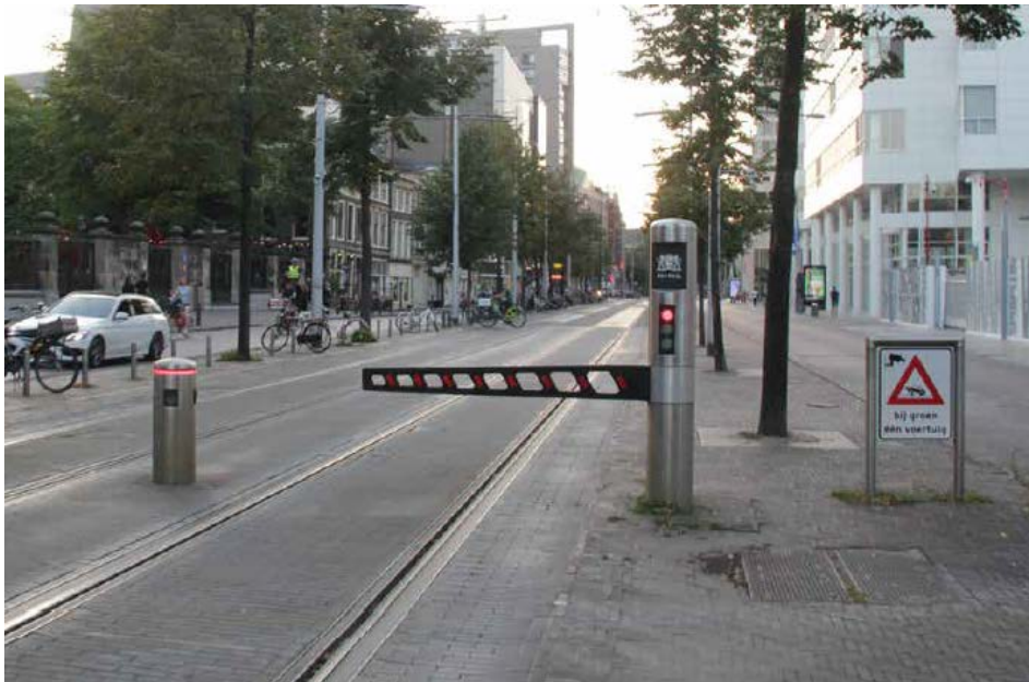
Figure 18. Example of automated gate in The Hague
