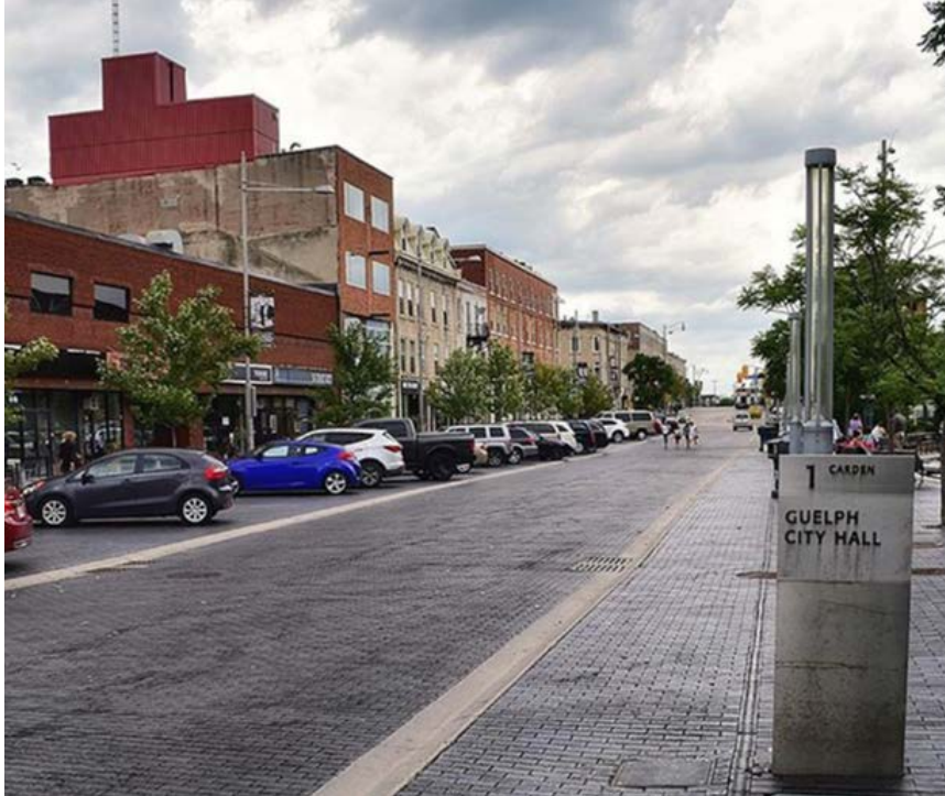
Figure 19. Example of mountable curb in Guelph, Ontario.
