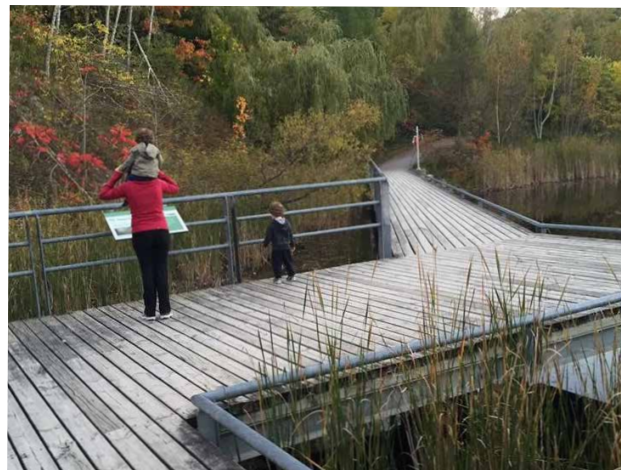
Deck Lookout with Elevated Platform
