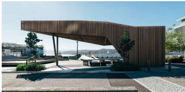
Pavillion Structure with Canopy
