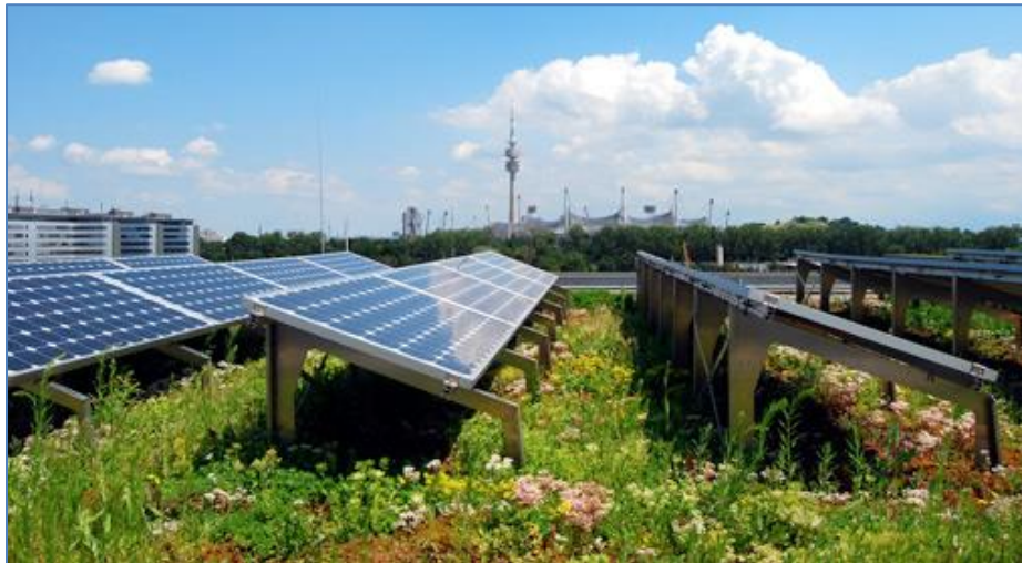
Figure 3. Solar PV installation on a green rooftop installation 1 .
