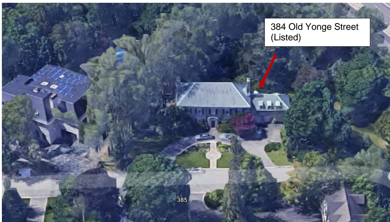
Figure 8. Google aerial view showing the similarities in typology & architectural styles between 324 Old Yonge Street and 384 Old Yonge Street (Listed)
