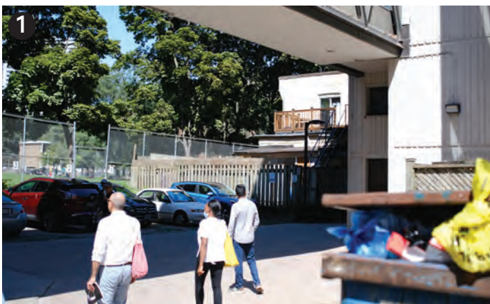
Walkway under Bridge of Fieldstone Co-Op
