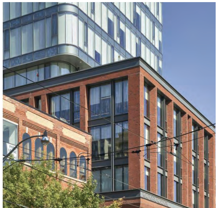
Figure 9: Masonry cladding at the podium level to complement existing heritage context.
