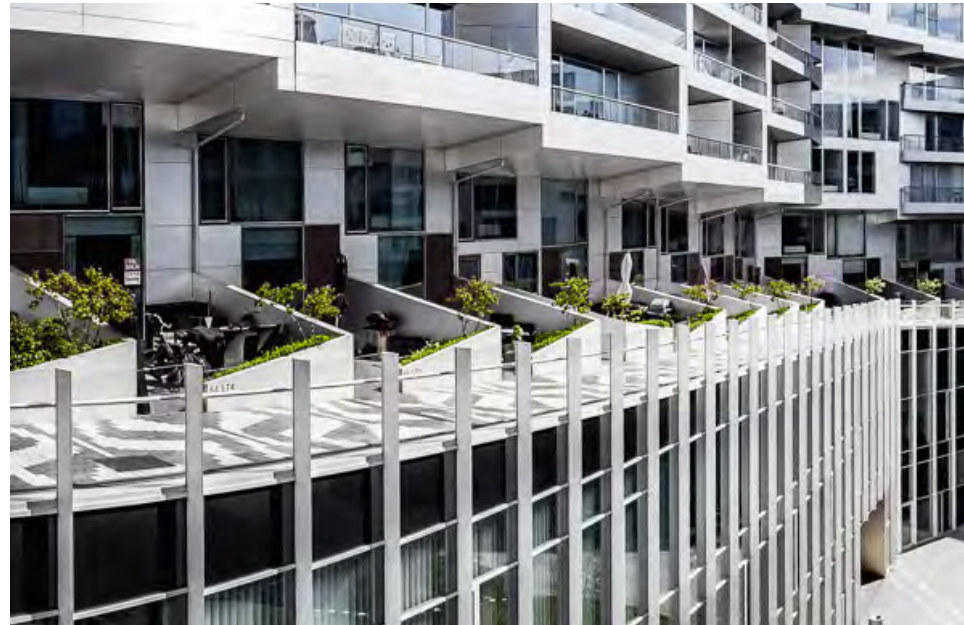
Tallet 8, Copenhagen - BIG Architects
