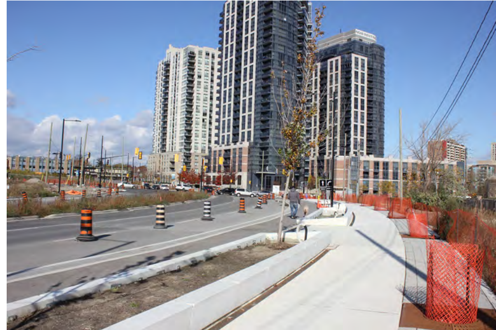
Dundas Street West - Looking Northeast (Block 3 & 6)
