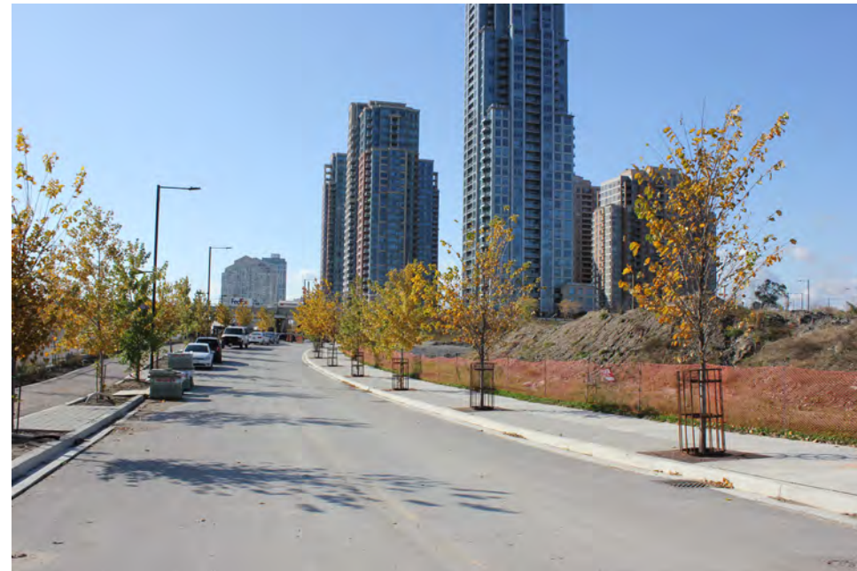
Road A Looking West (Block 1)
