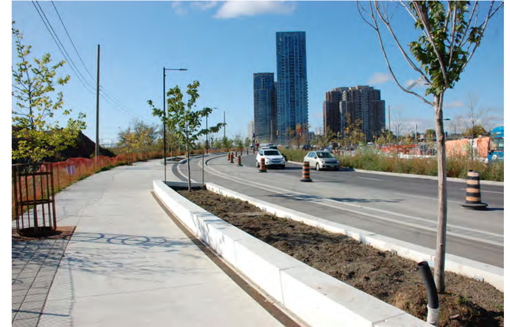
Dundas Street West - Looking Southwest (Block 3)
