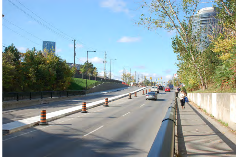
Bloor Street West - Approach to Site from East (Block 7)
