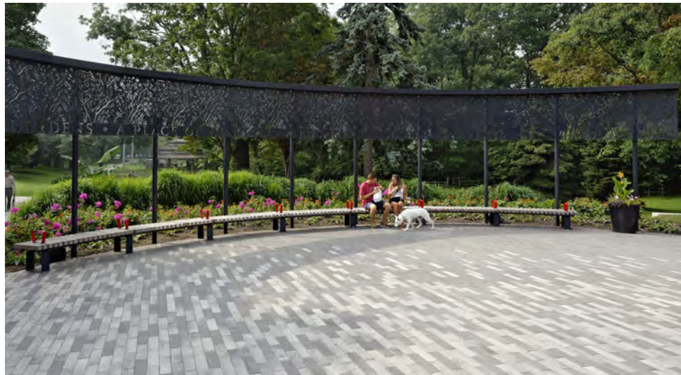
Architectural Screen, Kew Gardens Streetscape | Toronto
