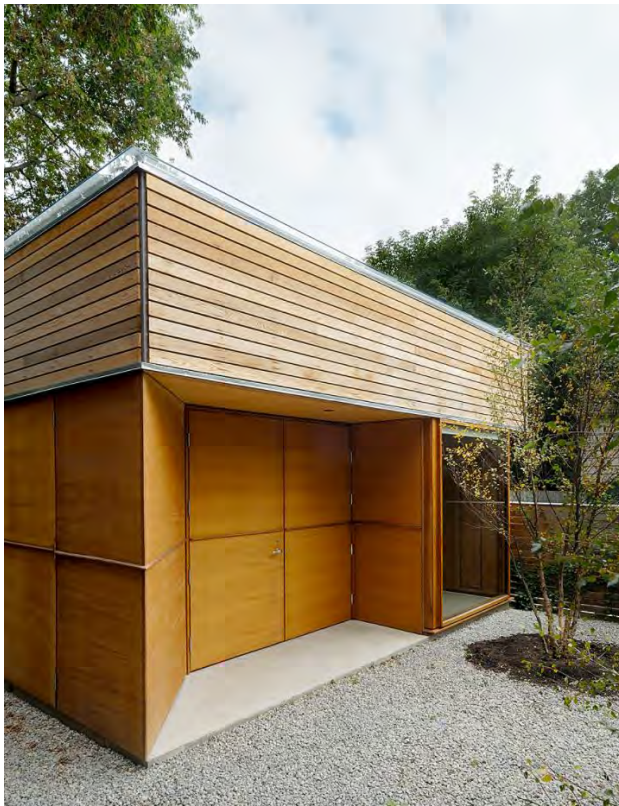
Craven Road Studio, 2004-6, Principal West elevation (Bob Gundu, RAIC, Architecture Canada 2010: Governor General's Medals , p.91)
