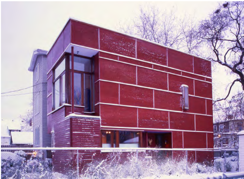
Figure 39. Craven Road House, west and south elevations with the effects of snow (Photo credit: Robert G. Hill)
