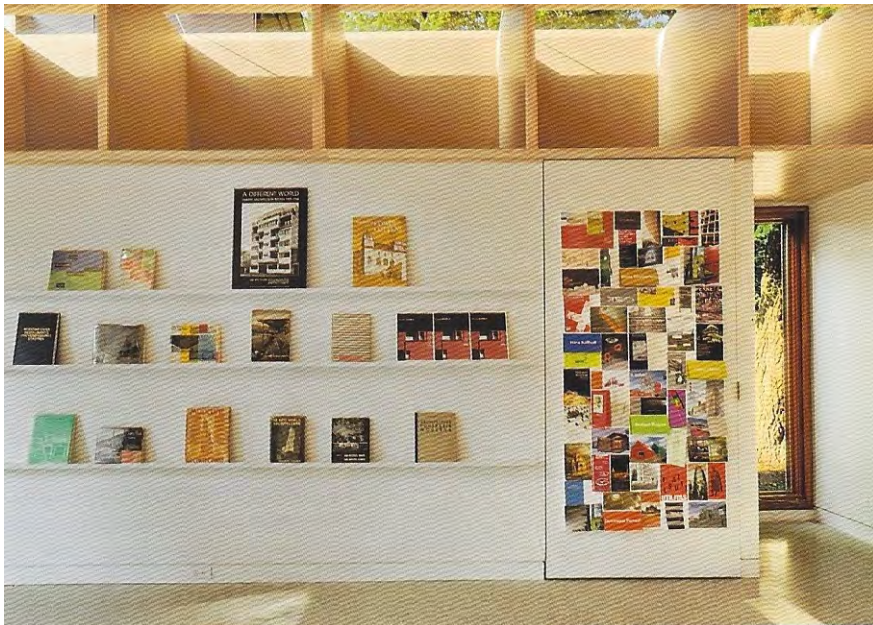
Figure 61. Studio Interior, north wall showing the deep coffers and their broad spacing with the display shelving below and the single window with a view of the rear garden and providing cross ventilation. (Photo credit: Bob Gundu, RAIC, Architecture Canada 2010: Governor General's Medals , p. 93.)
