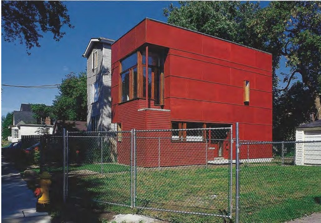
Figure 38. Craven Road House, west and south elevations, showing the street context with the adjacent three-storey house to the north and the row of cottages beyond and the garage to the south and its vacant land. (Photo credit: Michael Awad, Canadian Architect , July 1998, p. 24.)
