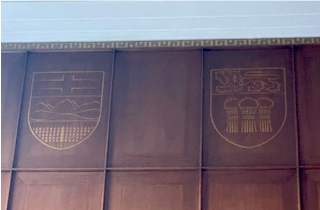
Figure 25: 250 University Avenue, entrance lobby, provincial crests with gold leaf gesso meander detail. Heritage Planning, 2021.
