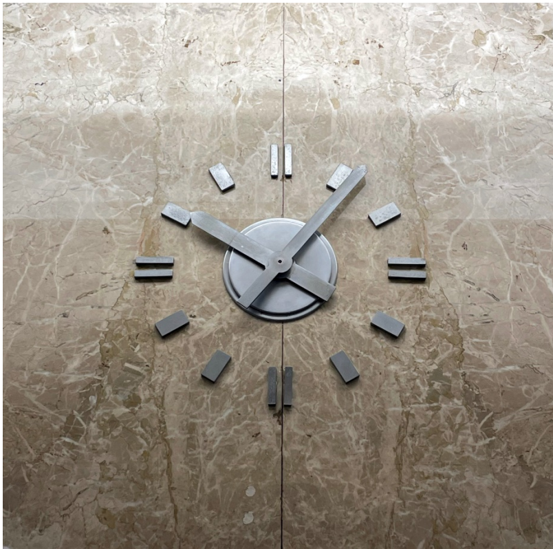
Figure 30: 250 University Avenue, elevator lobby, integrated clock detail. Heritage Planning, 2021.
