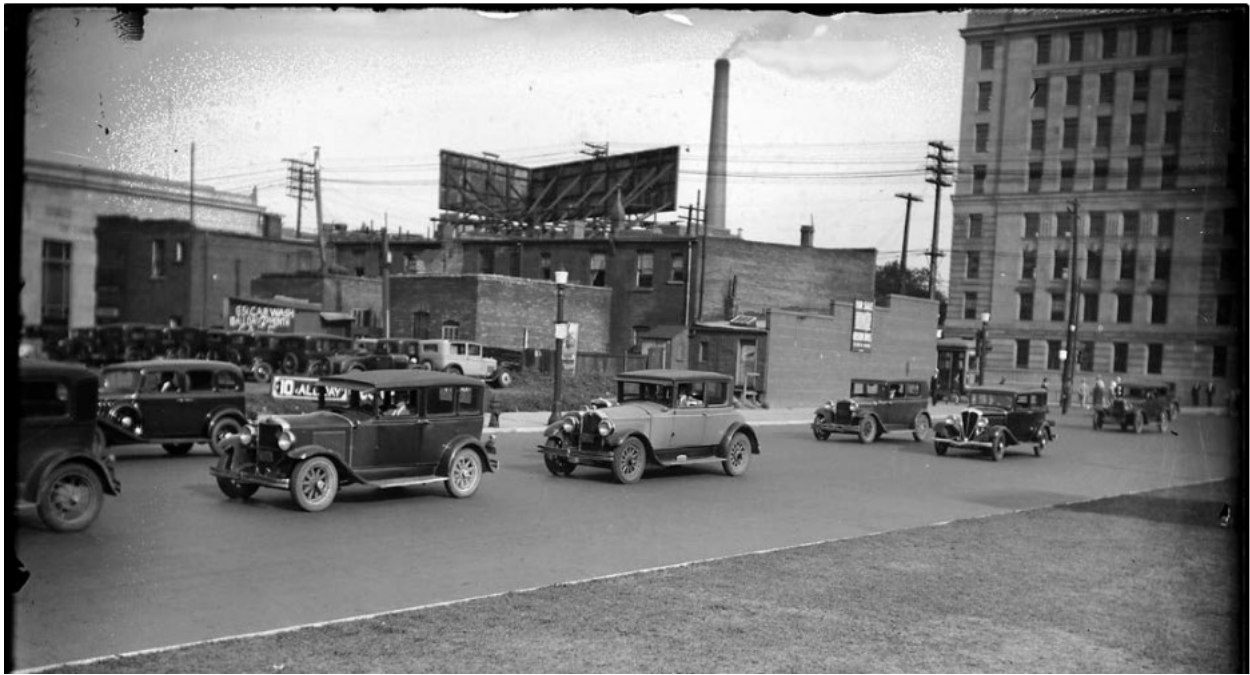
Figure 4: University Avenue, south of Queen Street West looking northwest showing the subject property prior to construction, 193- (City of Toronto Archives, fonds 1257, series 1057, item 31)
