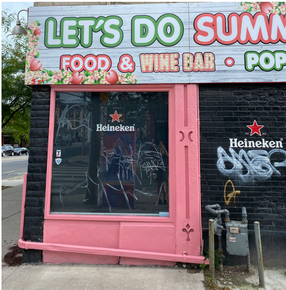
Figure 23: 164 Bathurst Street; detail of storefront glazing on north elevation; original or early wood pilaster visible at centre-right. (Heritage Planning, 2021.)
