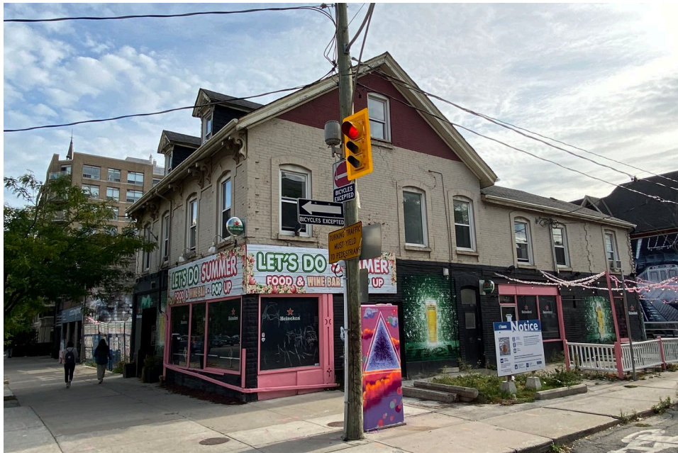
Figure 2: 164 Bathurst Street; southwestward view of the building's northeast corner, showing the north elevation along Richmond Street West. (Heritage Planning, 2021.)
