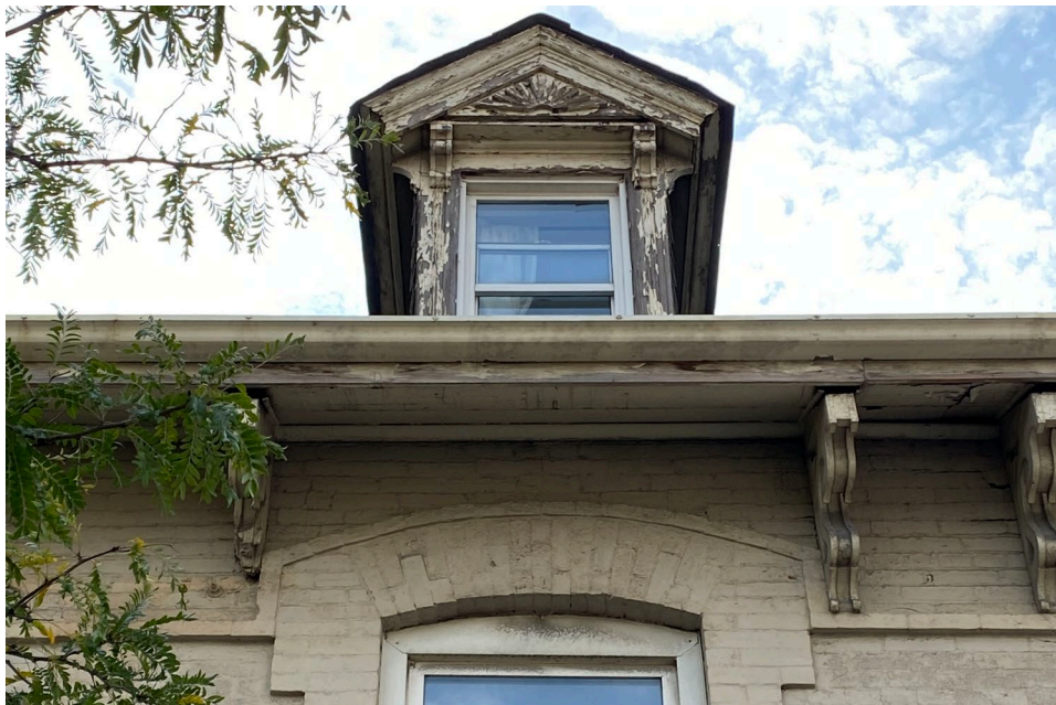
Figure 22: 164 Bathurst Street; detail of segmentally arched brick window surround, wood brackets, and dormer ornamentation on east elevation. (Heritage Planning, 2021.)
