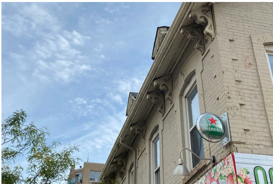
Figure 24: 164 Bathurst Street; detail of eaves and wood brackets on east elevation and quoins on northeast corner. (Heritage Planning, 2021.)
