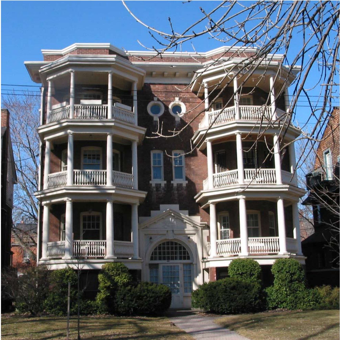
Figure 2: Principal (East) elevation of 68 Kendal Ave
