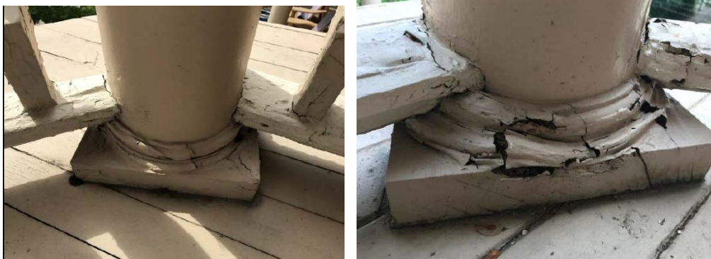
Figure 4-5: Deterioration at column bases
