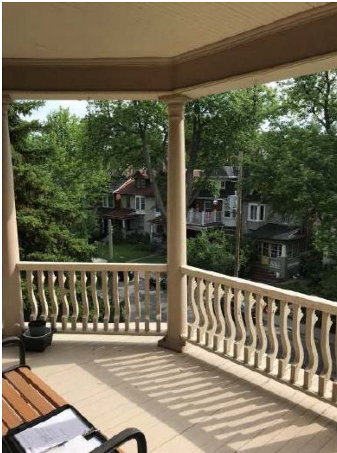
Figure 3: Typical view of balcony condition
