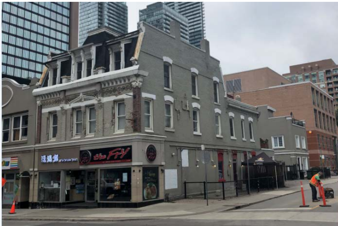
East (principal) and north (secondary) elevations of 526 Yonge Street at the southwest corner of Yonge and Breda Streets (Heritage Planning, 2021)
