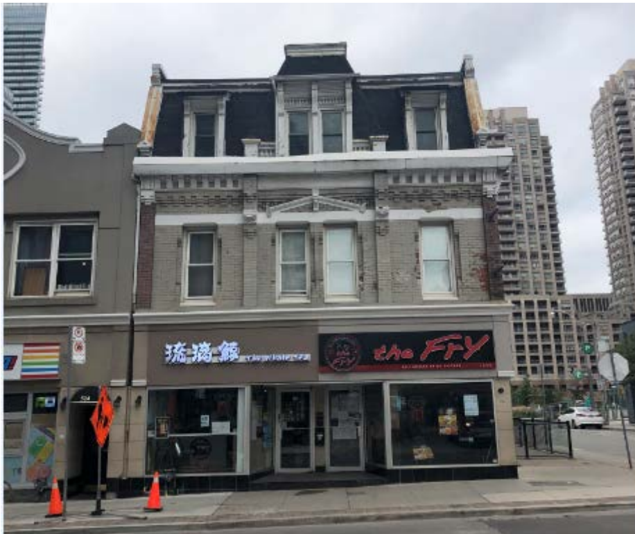
18. Current photo looking west, showing the principal (east) elevation of the building at 526 Yonge Street, located at the southwest corner of Yonge and Breadalbane Streets. (Heritage Planning, 2021)
