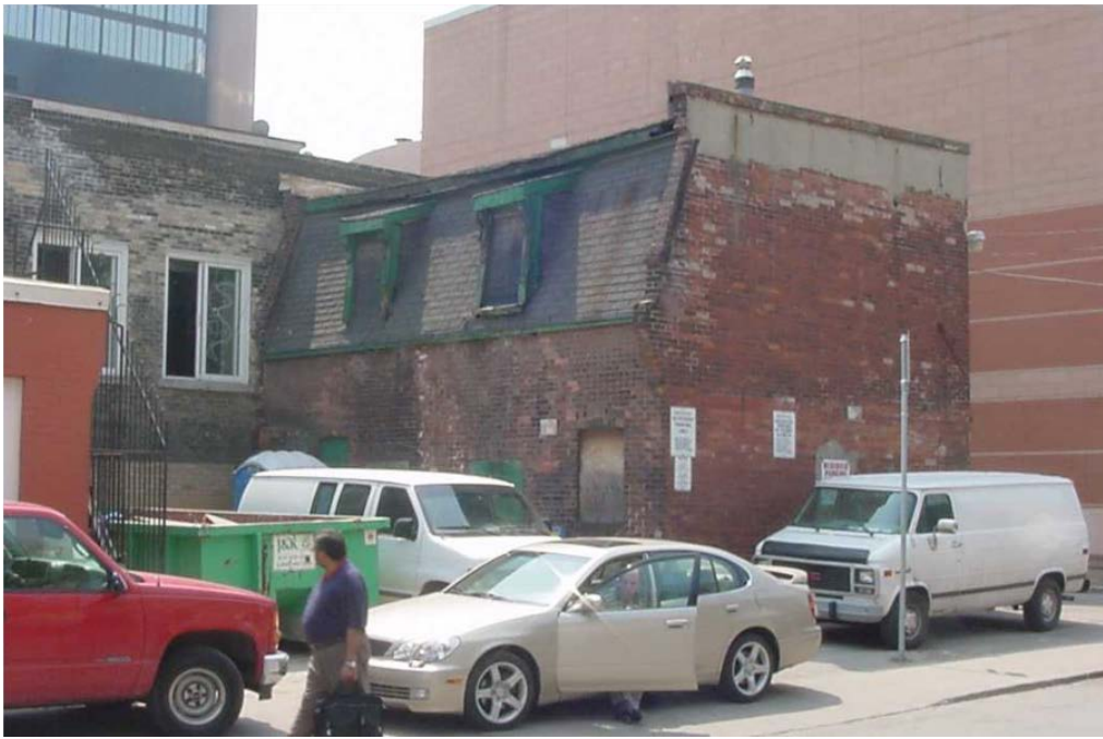
12. 2001 archival photograph, showing the rear coach house at 526 Yonge Street. Note this structure originally echoed the Second Empire design of the main building, featuring brick construction, and a mansard roof with shed-roofed dormers on brackets and parapet firewalls. (Heritage Planning, 2001)
