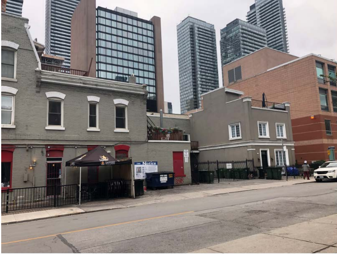
20. Current photo looking southwest from Breadalbane Street, showing the partial secondary (north) elevation of the building at 526 Yonge Street, and the coach house at the rear of the property, which underwent significant alterations in the early 2000s. (Heritage Planning, 2021)
