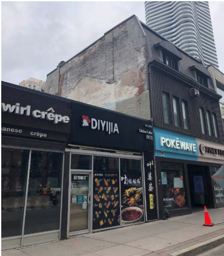
16. Current photograph looking northwest, showing the side (south) and principal (east) elevations of the building at 516 Yonge Street. (Heritage Planning, 2021)
