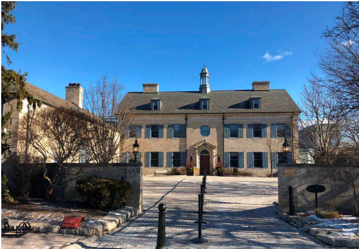
27. View of the walled forecourt with the principal (west) elevation of the house and the service-garage building to the left
