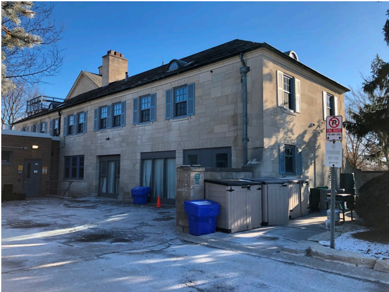
46. North and west elevation of the service-garage building with the gable of the main house beyond
