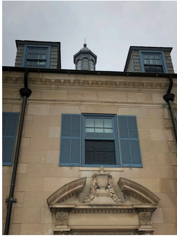
35. Photograph (above) showing the upper storey, dormers and cupola
