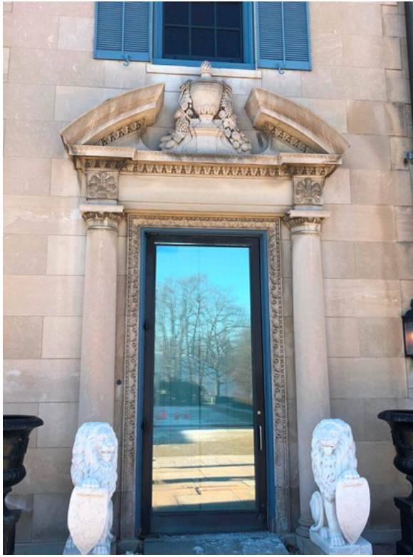
34. East elevation entrance from terrace (left)
