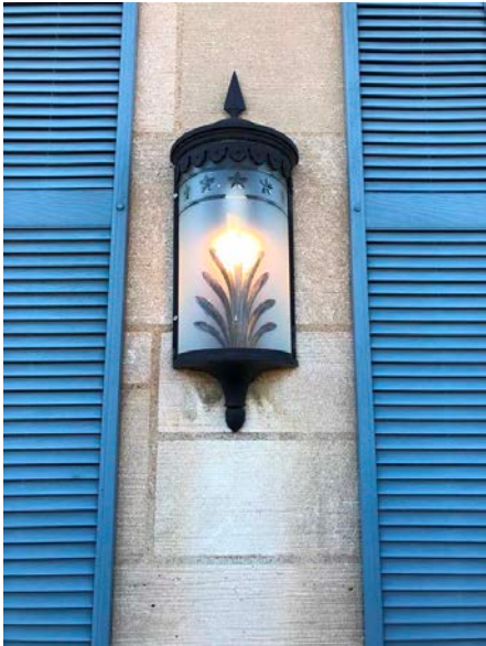
36. East elevation light fittings (left)
