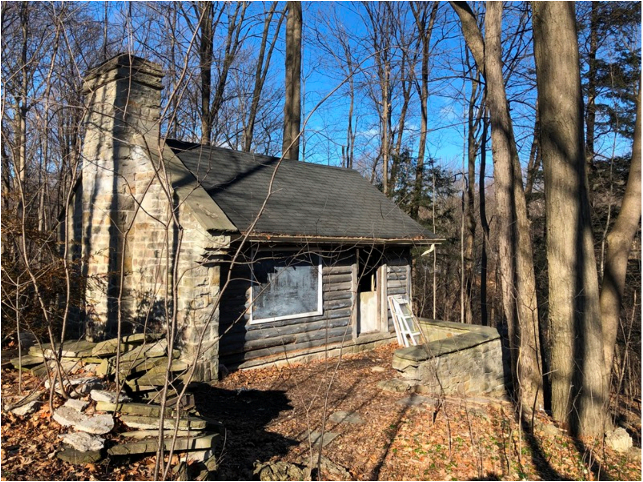
50. West and south elevations of the cabin showing the combination of west stone wall with chimney and log walls with stone terrace walls
