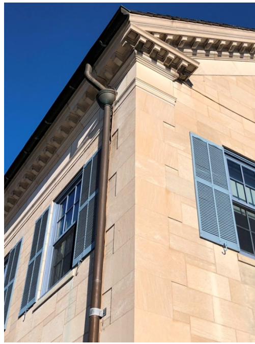
31. Photograph of the west entrance door case and octagonal window above 32. Photograph of the south-west corner of the house showing the stone details, quoins, entablature, cornice with returns and rain water leader
