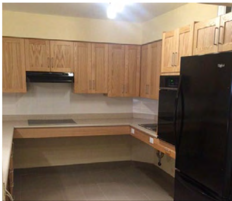
Kitchen modification showing lowered counter in a U shape, there are no cupboards underneath. A wheelchair user will be able to use all parts of the counter. There is a sink and a cooktop mounted on the counter.
