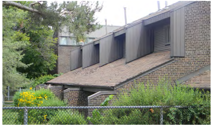
Example of multi-unit housing in the study area.
