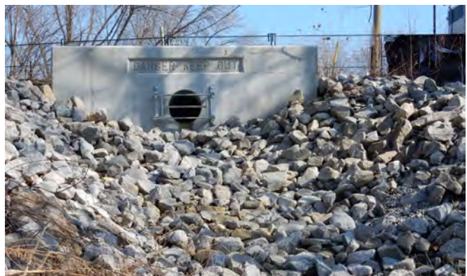
A stormwater outfall.
