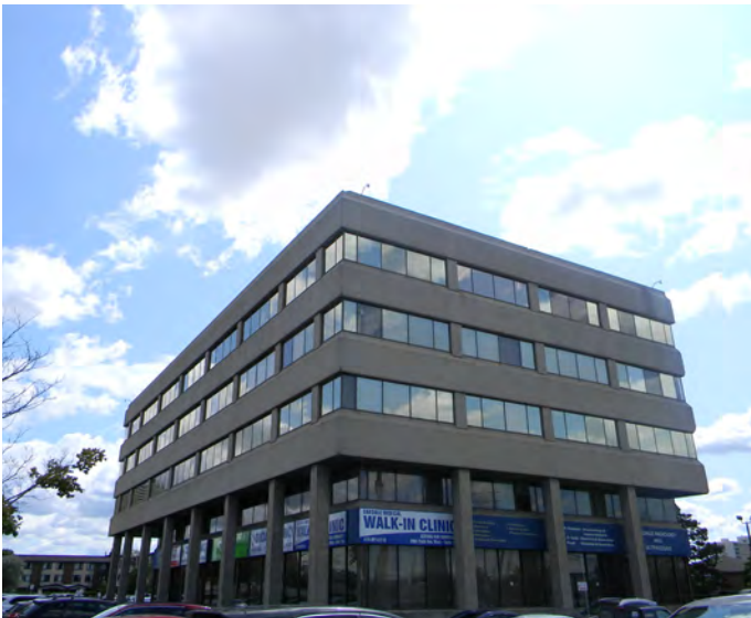
Medical services and other offices at the west end of Finch within the study area.
