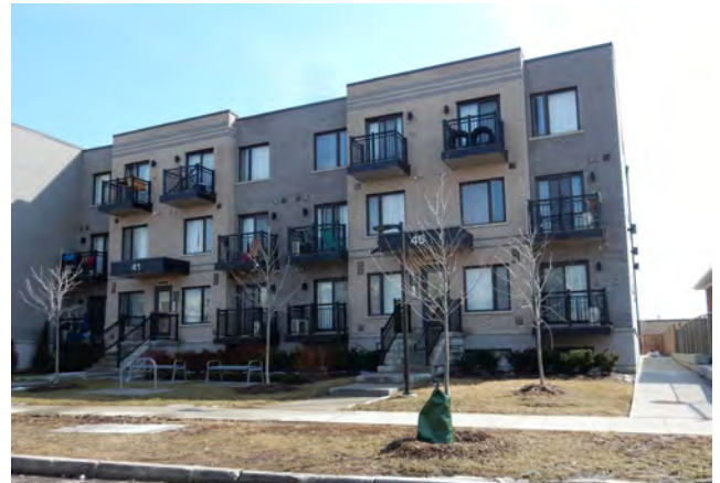
Example of multi-unit housing in the study area.
