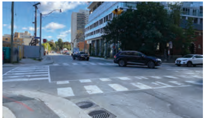
Figure 45 Existing condition at the intersection of Broadway Avenue and Redpath Avenue
