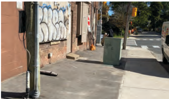
Figure 44 Existing condition at the intersection of Broadway Avenue and Mount Pleasant Road
