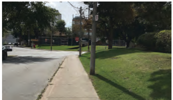
Figure 151 Existing conflicts with hydro poles along Pailton Crescent
