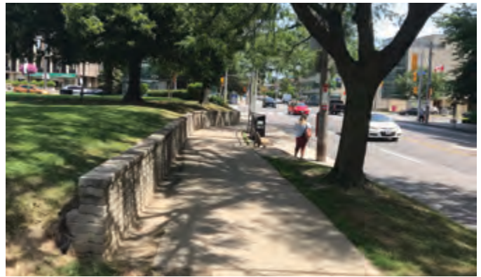
Figure 103 Existing retaining walls at June Rowlands Park
