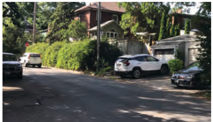
Figure 251 Missing sidewalk on the west side on Redpath Avenue, south of Soudan Avenue
