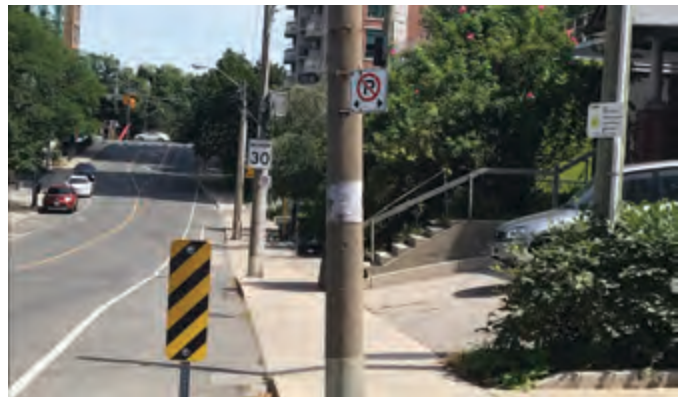
Figure 131 Existing hydro poles along Merton Street
