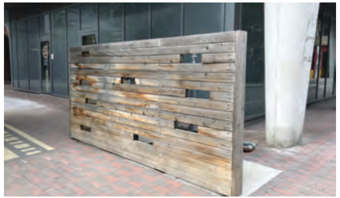
Figure 82 Transformer Screen at Adelaide Place
