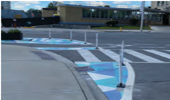
Figure 161 Painted bump-out at intersection with Yonge Street
