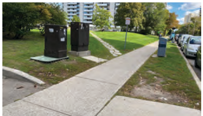
Figure 170 Existing utility conflicts along Balliol Street
