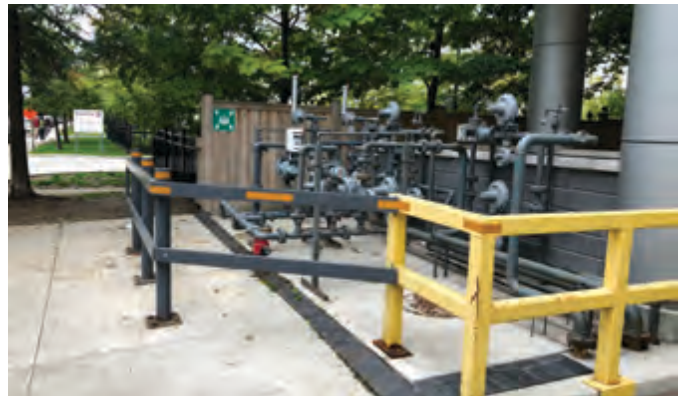
Figure 229 Utility conflicts along Lillian Street
