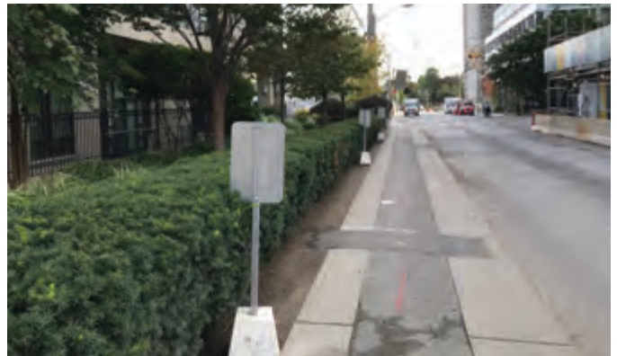
Figure 59 Constrained Condition at north west corner of Broadway and Redpath Avenues
