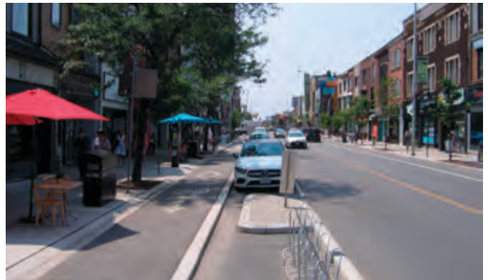
Figure 112 Raised Bikeway on Bloor Street
