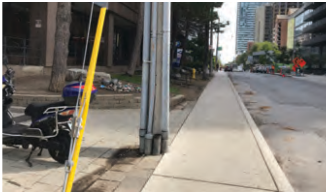
Figure 55 Utility Challenges along Roehampton Avenue
