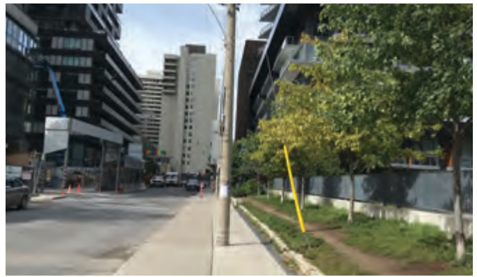
Figure 57 Utility Challenges along Roehampton Avenue
