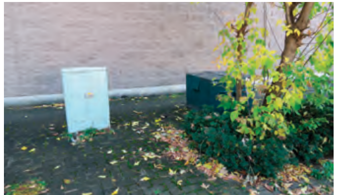
Figure 278 Utility challenges at Blythwood Road
