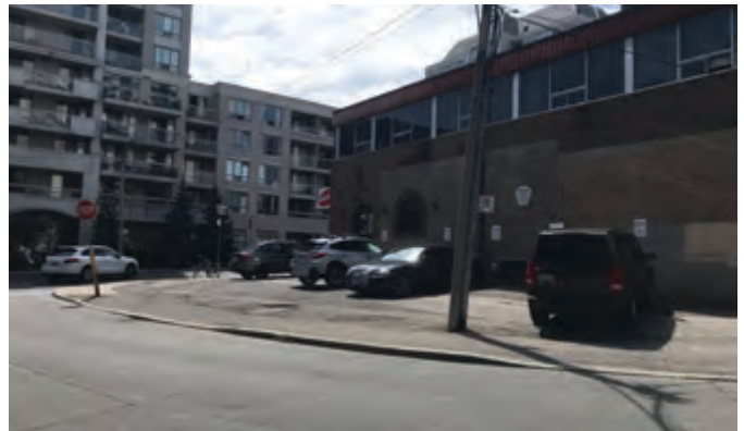
Figure 143 Existing condition with no sidewalk along west side of Pailton Crescent
