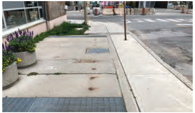
Figure 227 Utility conflicts along Brownlow Avenue
