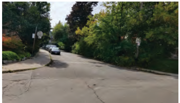
Figure 242 Existing condition south of Soudan Avenue on Redpath Avenue
