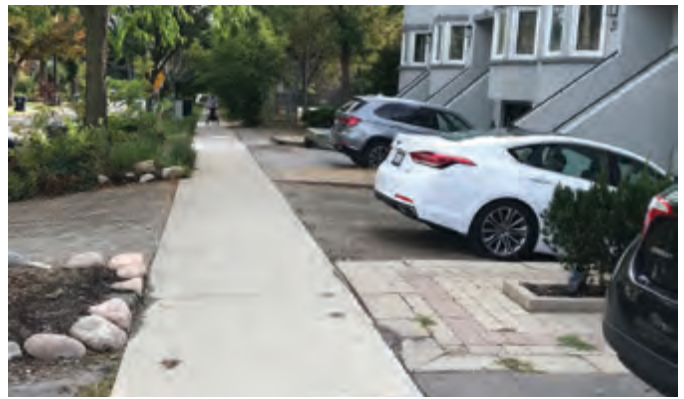
Figure 178 Existing condition along Keewatin Avenue
