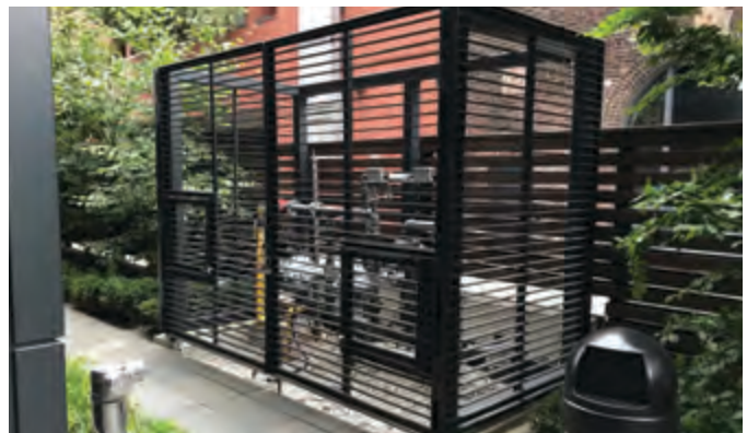
Figure 27 Transformer Screening, Sorauen Avenue
