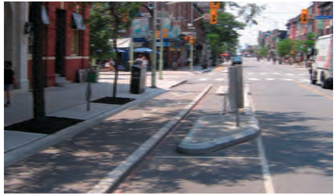
Figure 18 Raised cycle lanes on Bloor Street West
