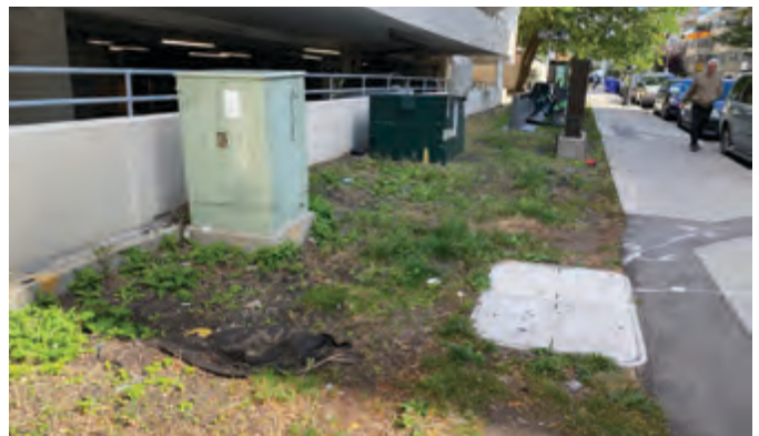
Figure 169 Existing utility conflicts along Balliol Street
