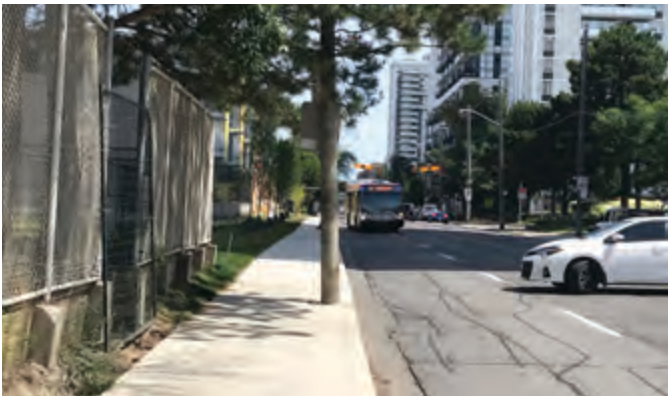
Figure 108 Existing utility conflicts along Davisville Avenue
