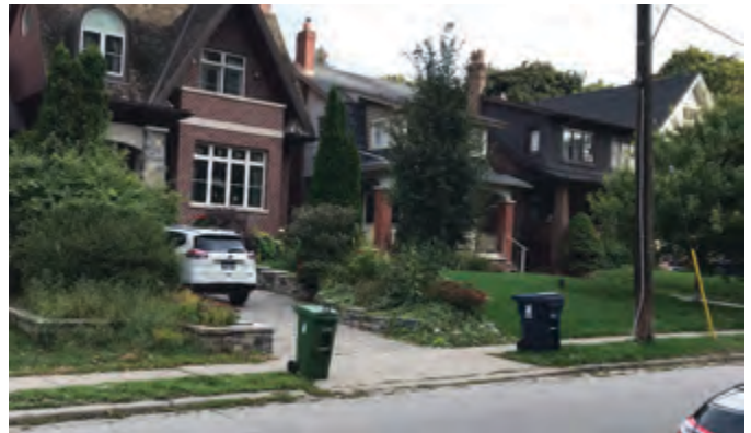
Figure 194 Existing garden walls along north side of Keewatin Avenue
