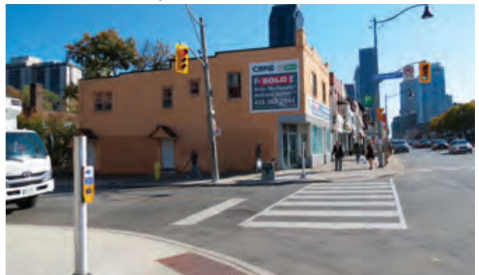
Figure 280 Heritage Building at Sherwood Avenue and Yonge Street
