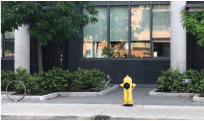
Figure 107 Existing fire hydrants along Davisville Avenue
