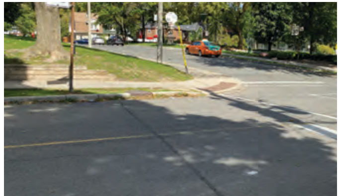
Figure 168 Existing grading challenges along Balliol Street
