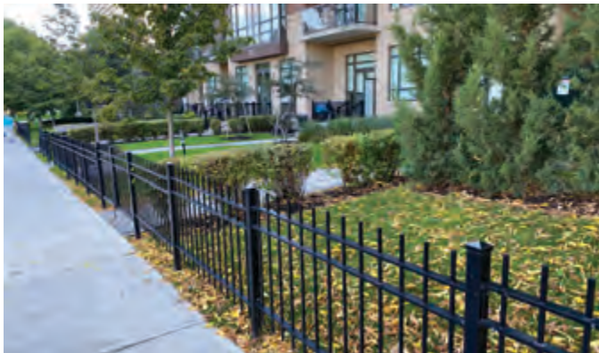
Figure 191 Existing fencing along Keewatin Avenue
