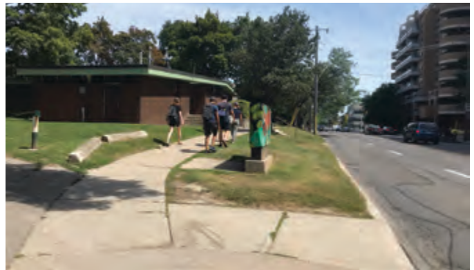
Figure 105 Existing sidewalk transition at June Rowlands Park
