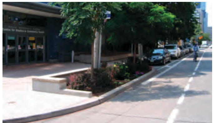
Figure 20 Bump-out at Gerrard and Mutual Streets
