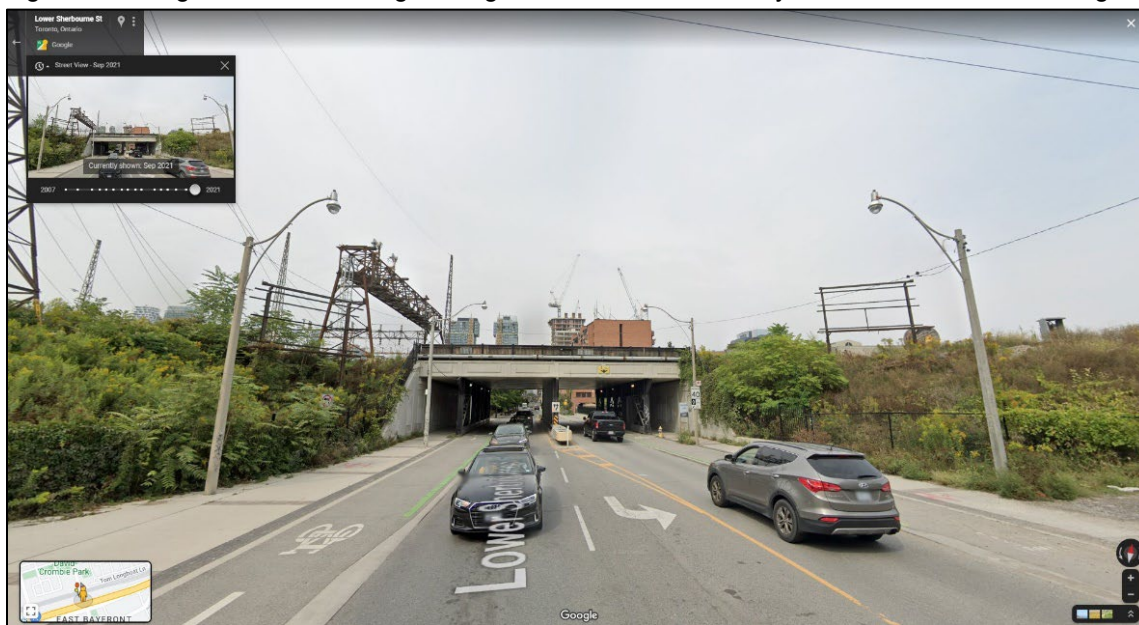
Figure 7 - Google Streetview image of Sign structures immediately south of the location of Sign 3
