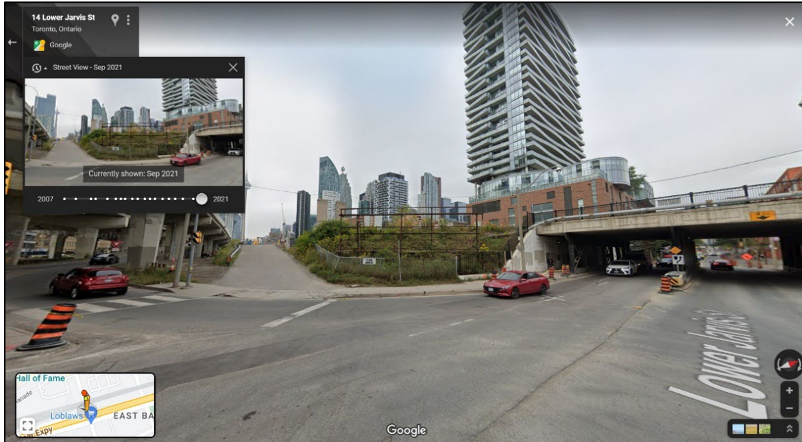
Figure 8 - Google Streetview image of a Sign structure at Lake Shore Blvd and Lower Jarvis Street
