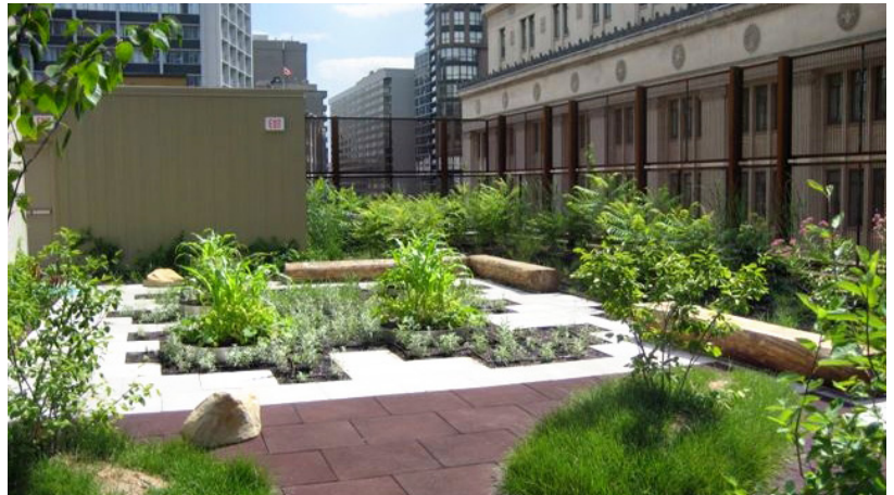
Traditional medicines, food crops, and native flowers, plants and grasses, are prominent features of the new green roof installed by Native Child and Family Services of Toronto.
