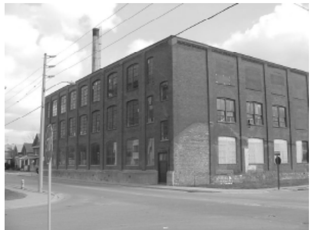
Source: Economic Development Services Branch, City of Oshawa An older building in Oshawa that has been purchased to develop live/work spaces.
