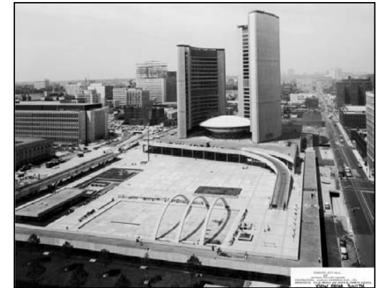
View from South: Construction Completed 1965
