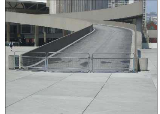
Ramp to Podium Level
