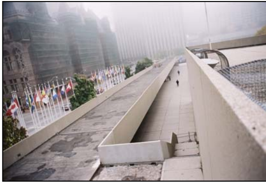
View from the podium level
