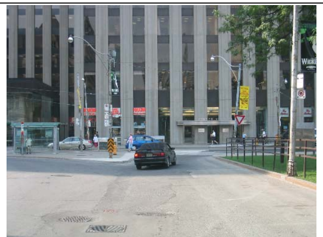
Southbound approach to right turn lane
