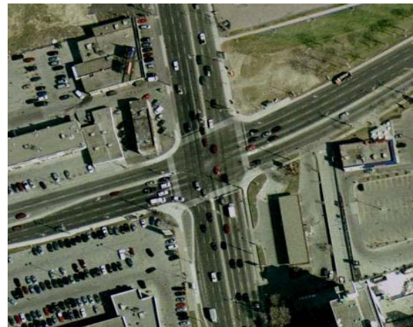
Figure 35 - Keele Street and Wilson Avenue intersection
