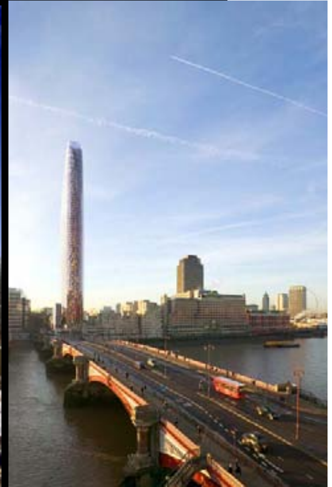
Blackfriars Bridge – Beetham Tower
