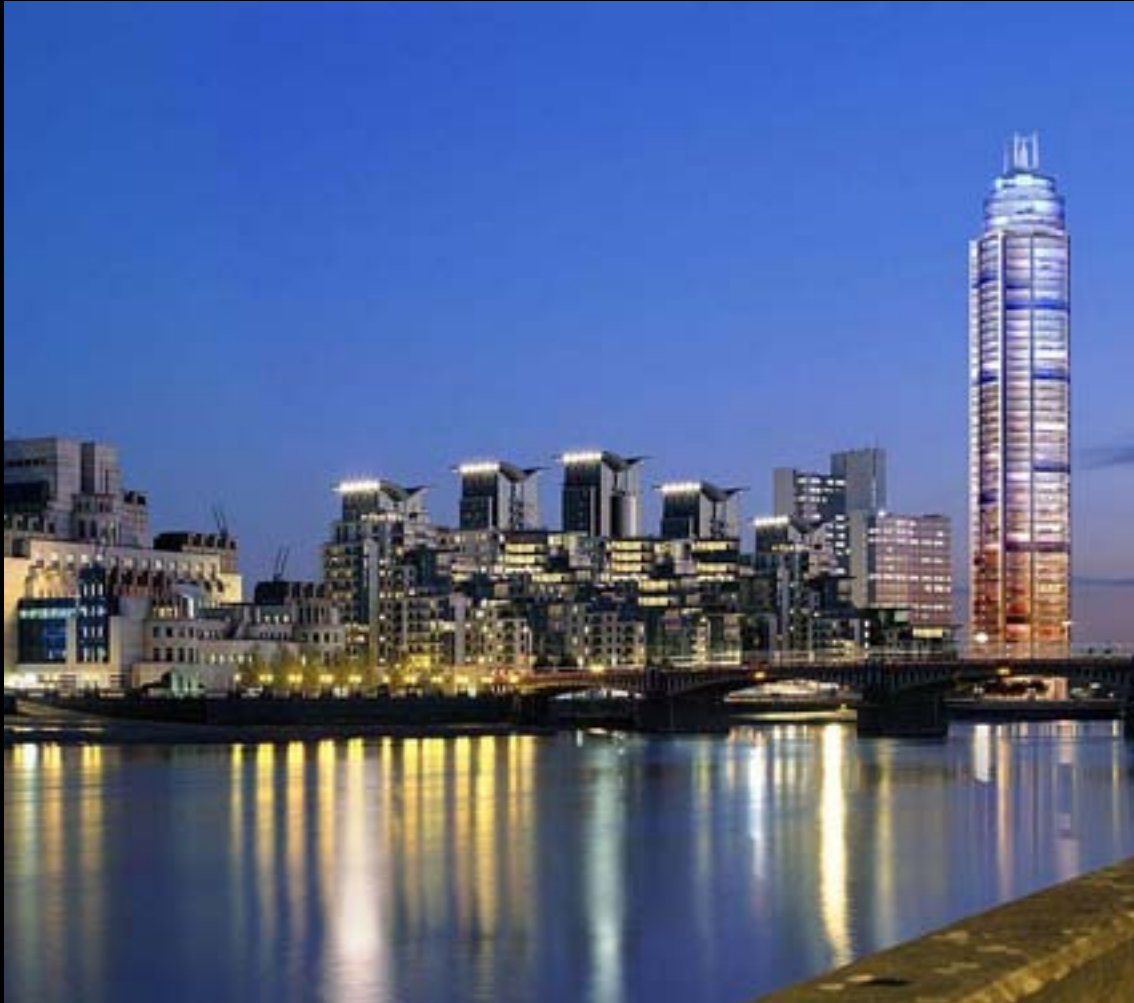
Vauxhall bridge tower
