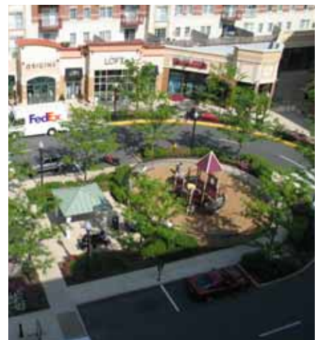
Precedent image highlighting high quality building design and mixed-use development to generate an active public realm
