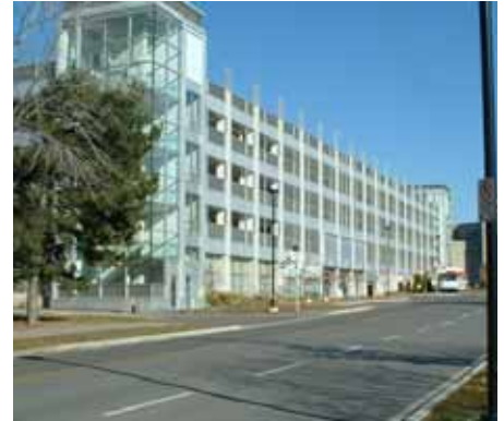
Precedent image highlighting how structured parking garages can be designed to fit with surrounding development
