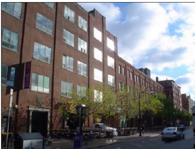
Photo 4 – Consistent street wall on The Esplanade
