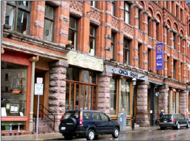
Photo 7 – Existing commercial buildings on Colborne Street
