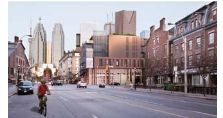
West View of the Gateway Framing the Gooderham Flat Iron Building
