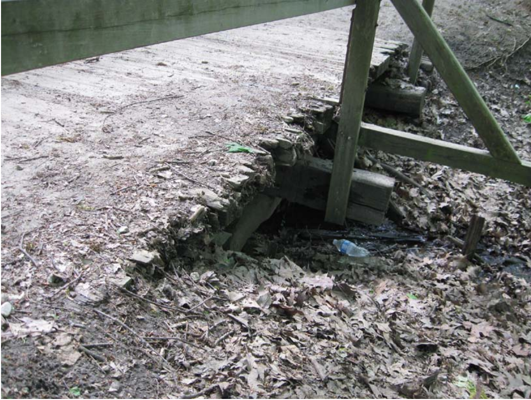
Existing condition of pedestrian bridges to be replaced.
