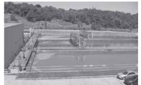
North primary tank
