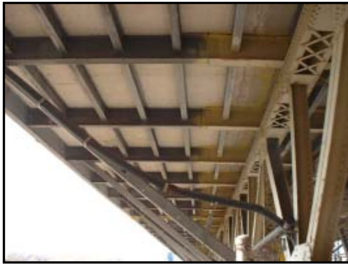
Existing Concrete Deck
