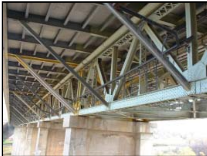
Existing Steel Structure
