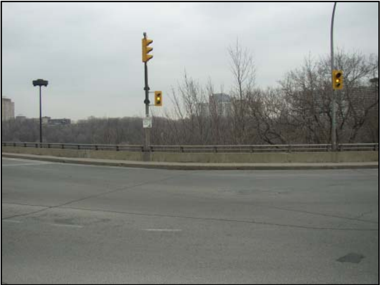
Existing Parapet Walls and Railing
