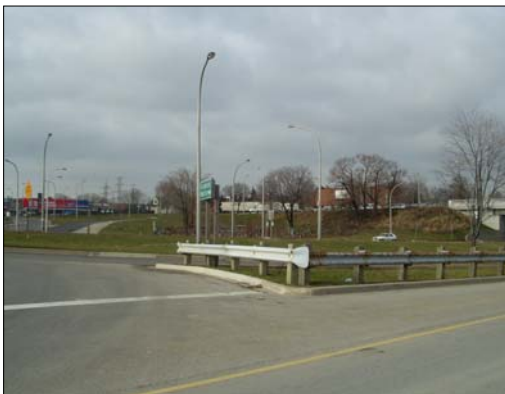
Facing northwest towards Six Points Interchange from the Kipling Avenue northbound ramp, east of Kipling Avenue.
