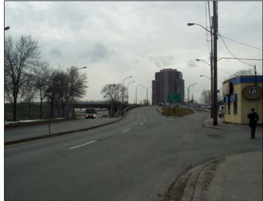
Facing southwest towards Six Points Interchange along Dundas Street.
