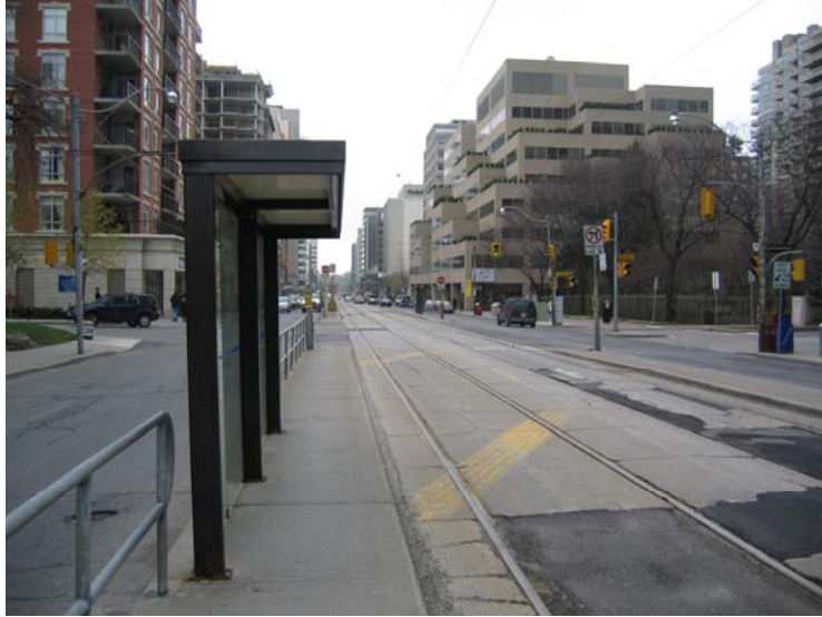
platform (existing condition)
