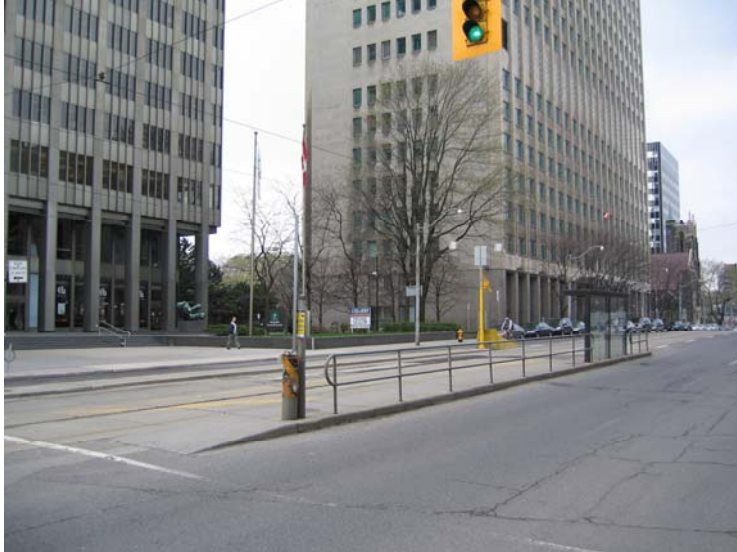
platform (existing condition)
