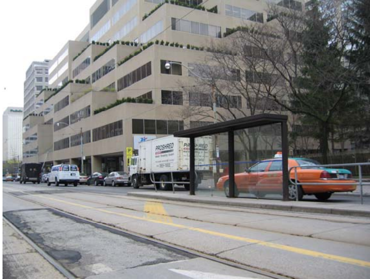
shelter (existing condition)
