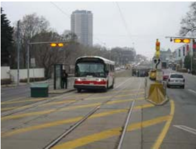
Ramp to tunnel at the St. Clair West subway station.
