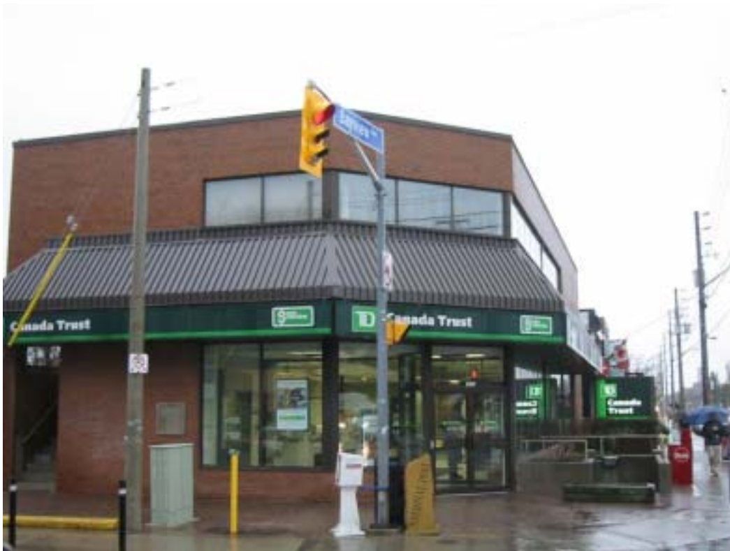
Corner of Bayview Ave. and Millwood Rd.
