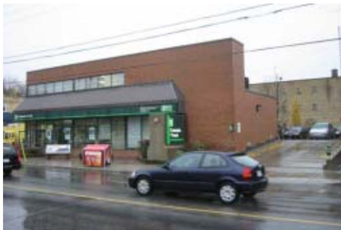
Bayview Ave. side.
