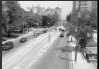
St. Clair Avenue at Avenue Road – existing conditions
