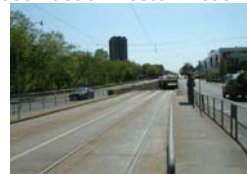
Underpass East of Weston Road
