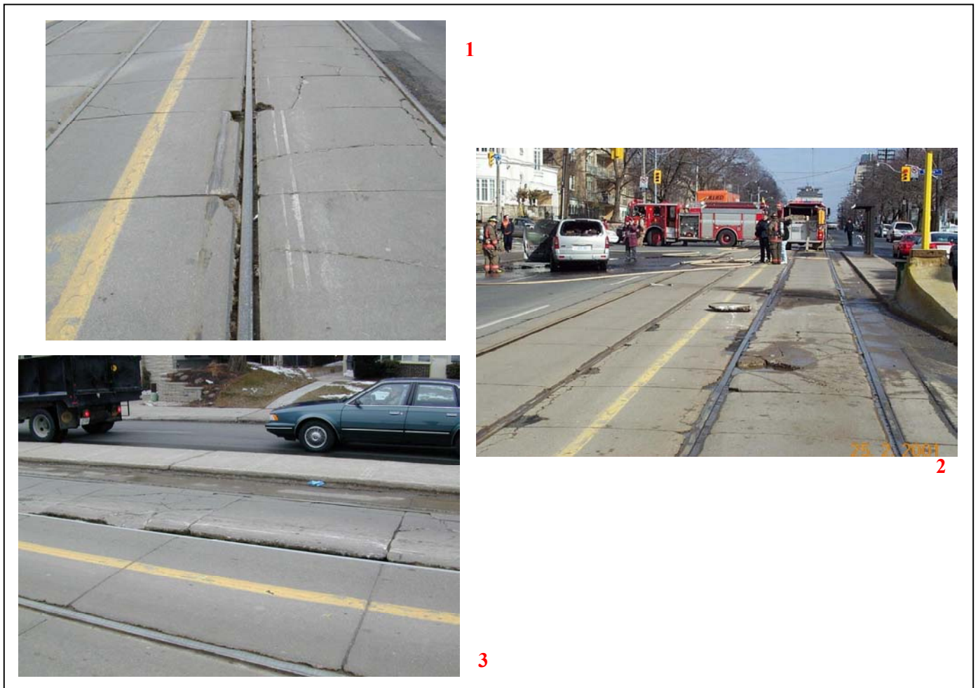
Figure 6.2.1: Photographs of the Existing Condition of the St. Clair Streetcar Trackbed
