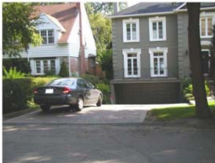
Reverse slope driveway with crown to mitigate flooding
