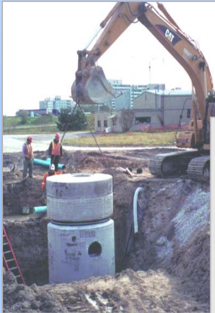
Typical Unit being Installed
