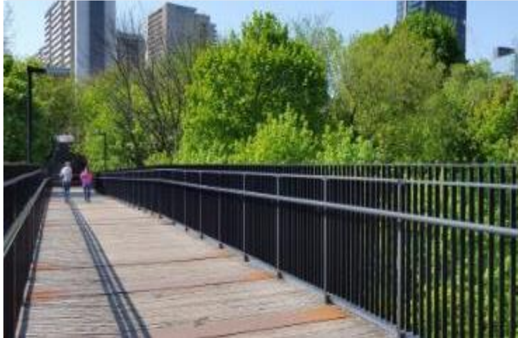
View on pedestrian bridge looking south
