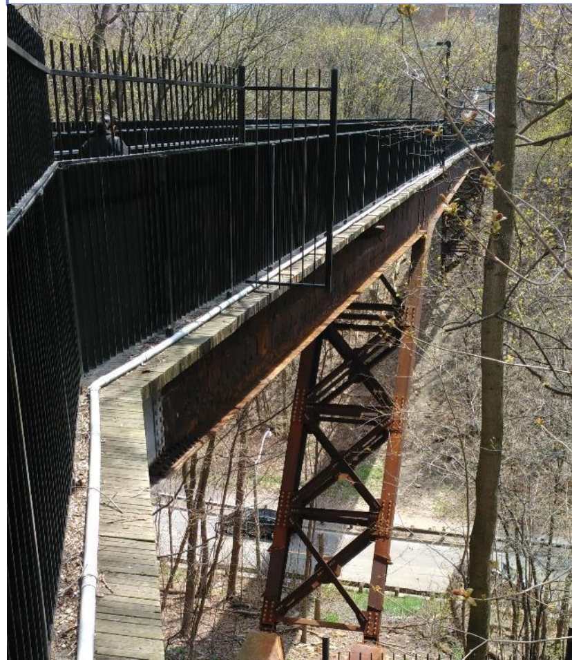
View on bridge looking south
