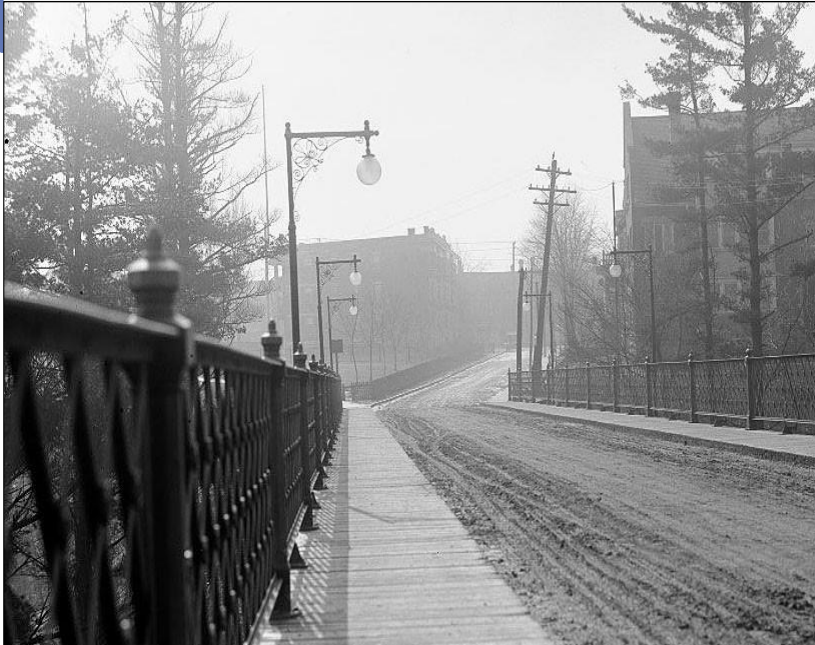
View of vehicular bridge looking south
