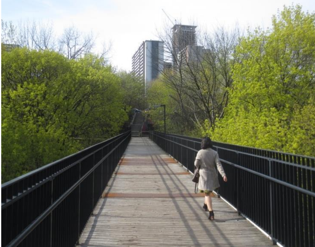
View from mid-bridge looking south
