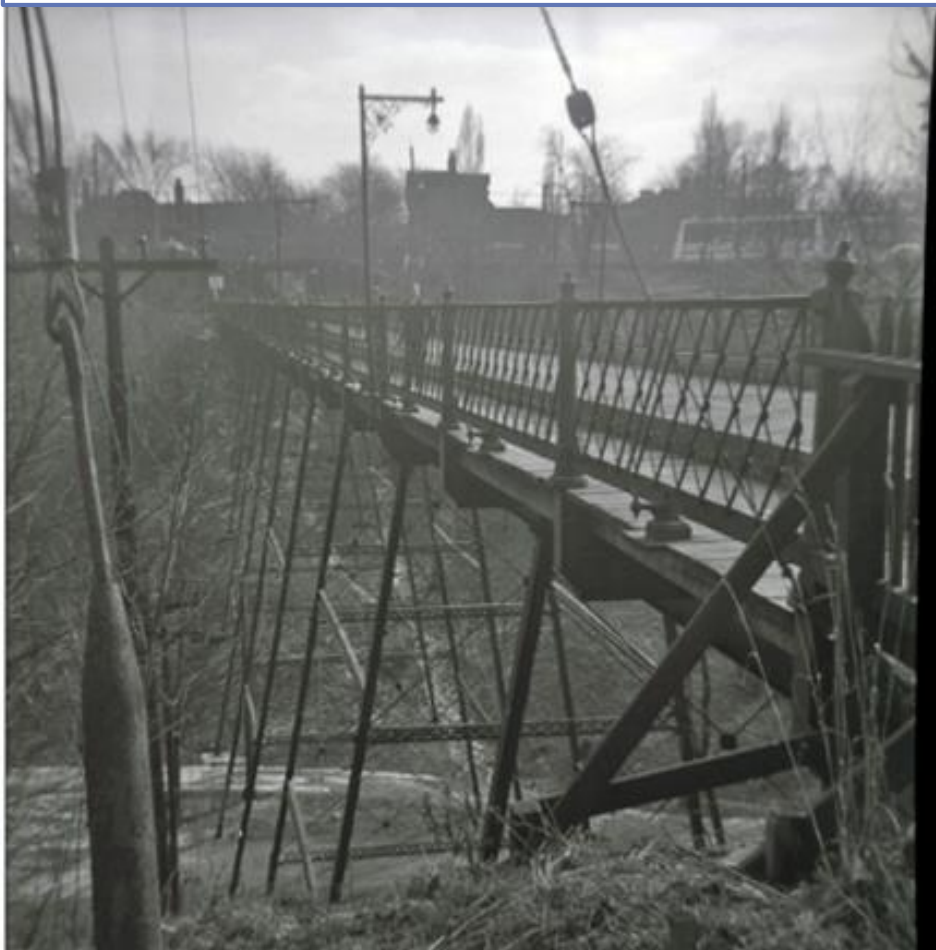
View of bridge looking south (1951)
