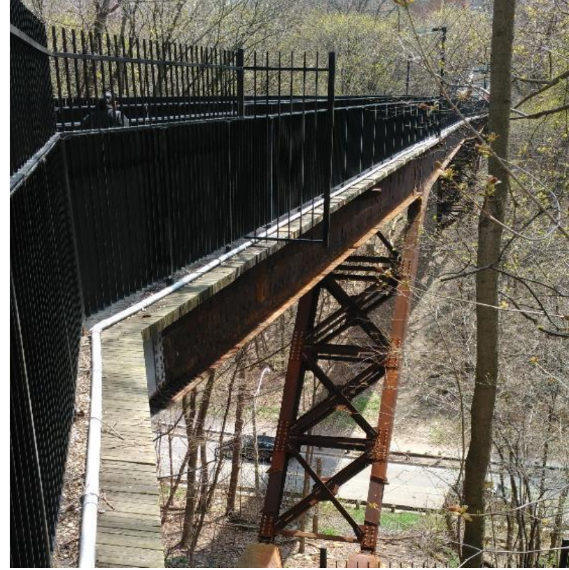
View from north abutment looking south
