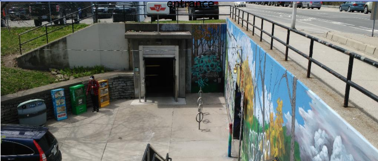
View from south side of Bloor Street East looking to tunnel and TTC entrance
