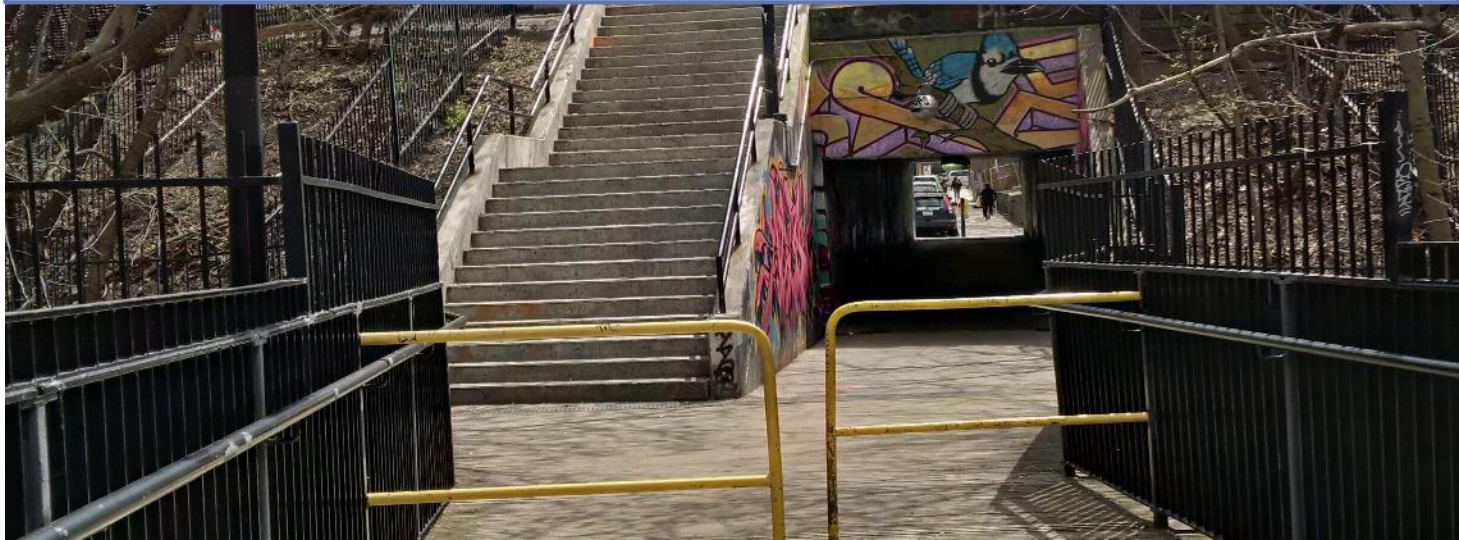
View from bridge to south approach and tunnel
