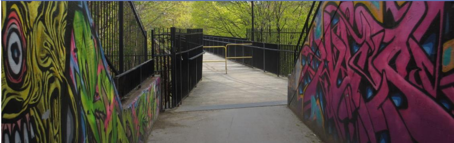
View from tunnel looking north to bridge
