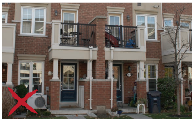
Example of a front facade over-cluttered with rainwater leaders, air conditioning units, utilities, and vents.
