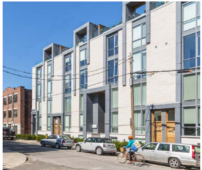
The hybrid building type can be employed when a reduction in individual unit access to grade is warranted.
