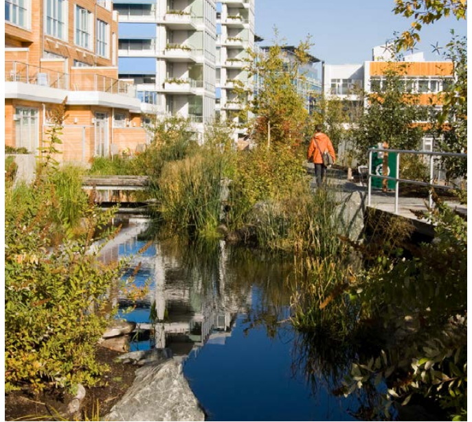
Bio-retention integrated into development. Credit: PWL Partnership Landscape Architects
