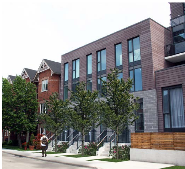
New townhouses transition in height and setback to fit-in with surrounding context.
