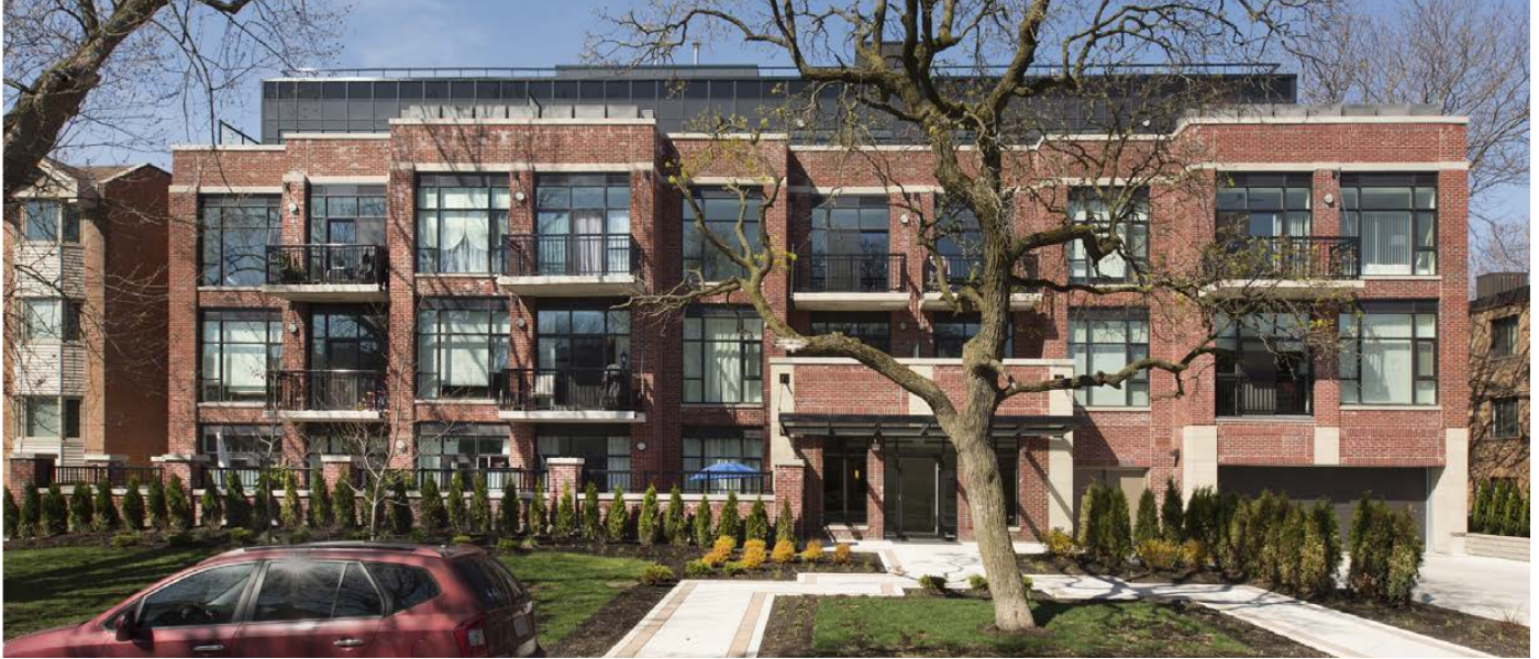
Public realm can be significantly improved when garage ramps and garbage storage areas are internalized into the building. Credit: Audax Architecture. Photo: Joy von Tiedemann.
