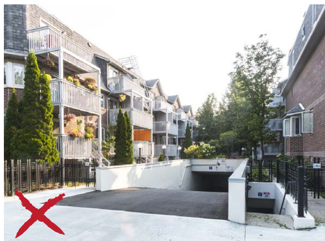
Avoid freestanding underground garage ramps and access stairs, incorporate within the building.
