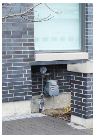
Locate and integrate utility meters in recessed coves and/or screen with landscape plantings to help maintain an attractive streetscape.
