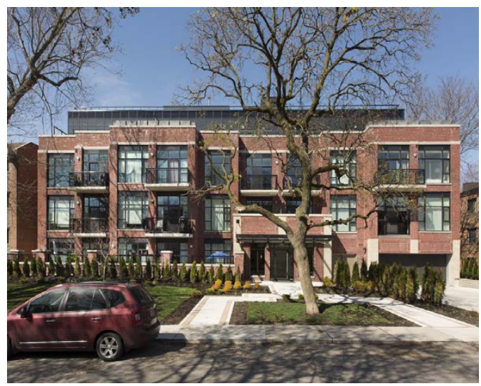
Low-rise apartment building fits into existing context. Credit: Audax Architecture. Photo: Joy von Tiedemann.
