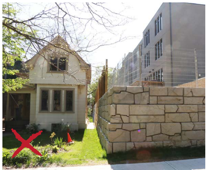
Grade alterations can create a negative impact on adjacent properties.
