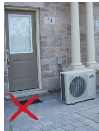
Poorly located utilities and mechanical systems adjacent to front entrance and street frontage negatively impact the quality and comfort of the public realm.
