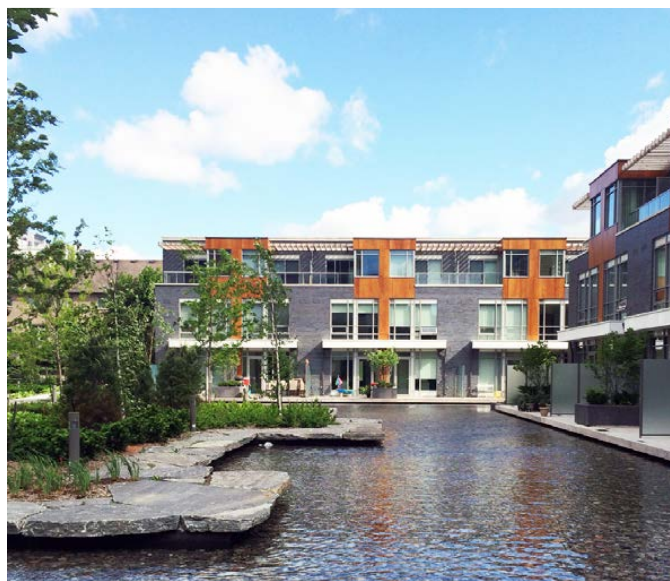
Townhouses frame a well-landscaped courtyard outdoor amenity area with reflecting pool.
