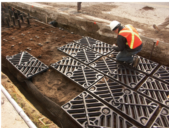
Figure 22 - Soil Cells. Queensway pilot project in collaboration with Toronto Water. Water from road and sidewalk diverted to soil cells from storm sewer and analyzed for quality.
